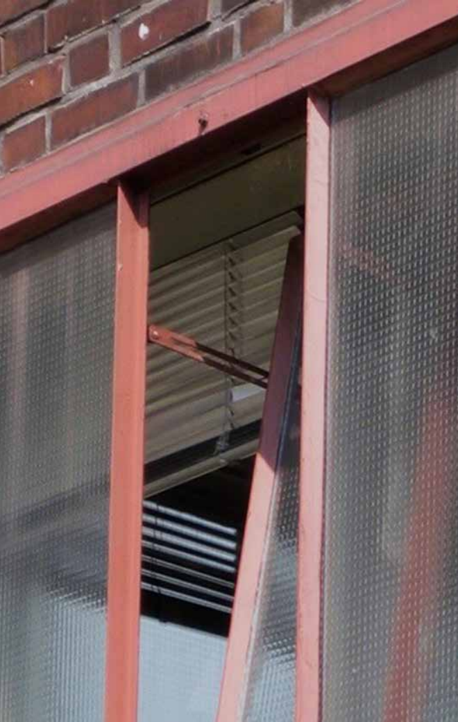
FIG. 5.21 Metal framed windows were used in industrial architecture since 18 th century, and became standard in 20 th century with mostly patterned or wired glass, Zollverein Coalmine, 1932 / Photo: U. Pottgiesser
