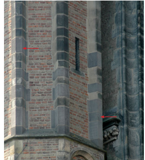
FIG. 2.9 Volvic basalt on the stair tower of the south transept of the Dom Church in Utrecht, as a replacement for Bentheim sandstone / Photo: W.J. Quist
