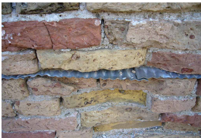
FIG. 3.4 Mechanical interruption of the wall by the use undulated steel sheets, Venice, Italy / Photo: R. van Hees
