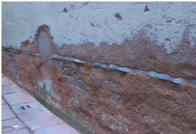
FIG. 3.3 Mechanical interruption of the wall by the use of plastic sheet, Venice, Italy / Photo: B. Lubelli
