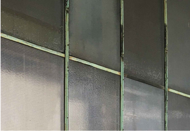
FIG. 5.9 Wire mesh glass, Lochal Tilburg / Photo: W.J. Quist
