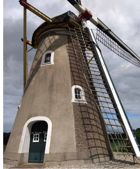
FIG. 4.10 A plaster layer for protection can be an alternative for a water-repellent treatment / Photo M. van Hunen
