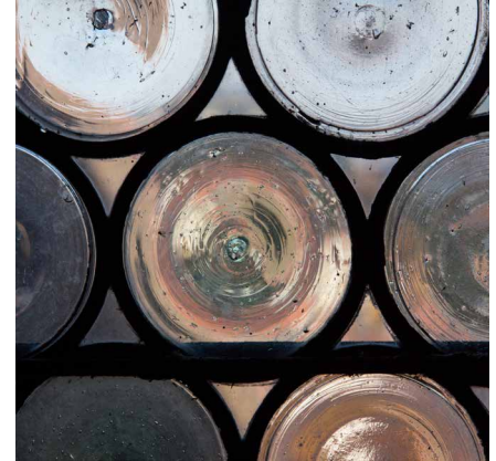
FIG. 5.4 Crown glass was one of the most common glass types until 19 th century / Photo: pixabay.com
