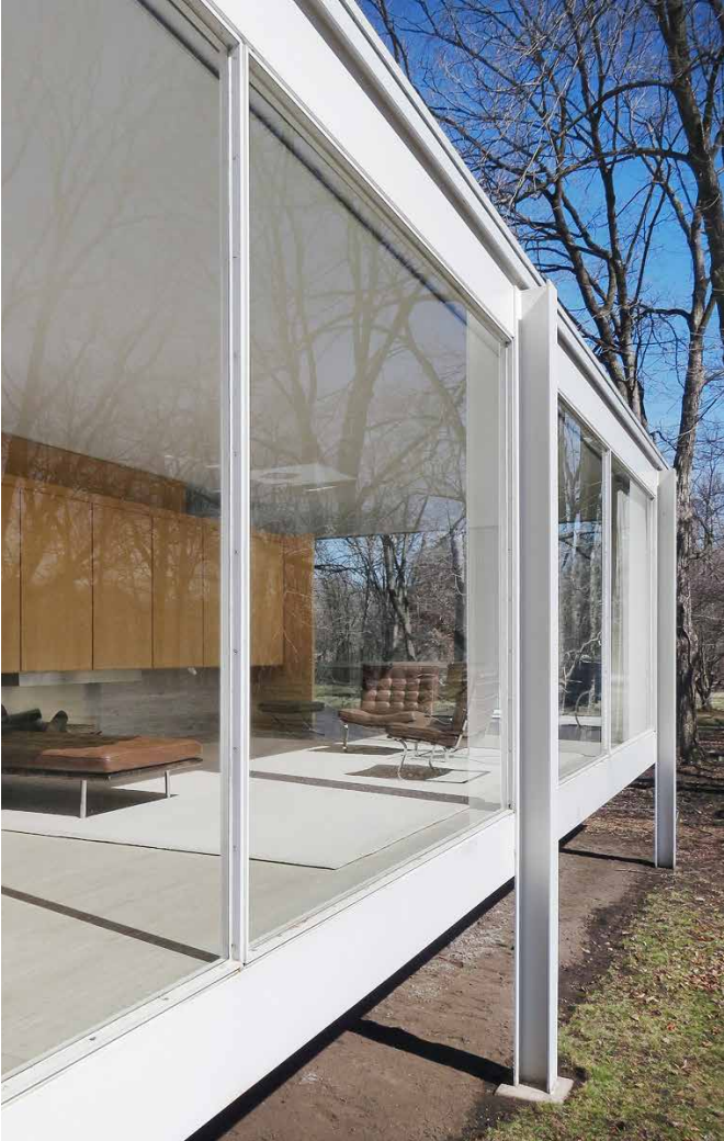
FIG. 5.22 Large metal framed windows were introduced to residential architecture in early 20 th century, and became famous with buildings like the Farnsworth House, 1951 / Photo: A. Ayón
