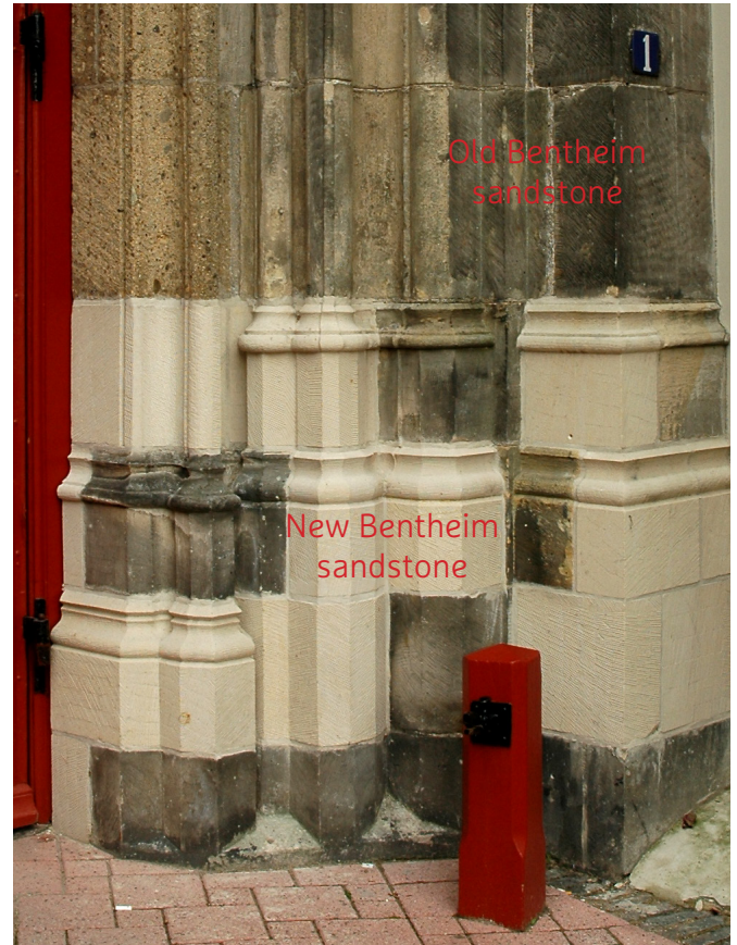
FIG. 2.11 Bentheim sandstone at the south portal of the Sint-Joriskerk Amersfoort / Photo: W.J. Quist
