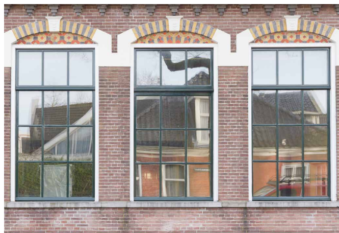
FIG. 5.17 Wooden window with muntins (glazing bars) connecting small glass panes / Photo: RCE
