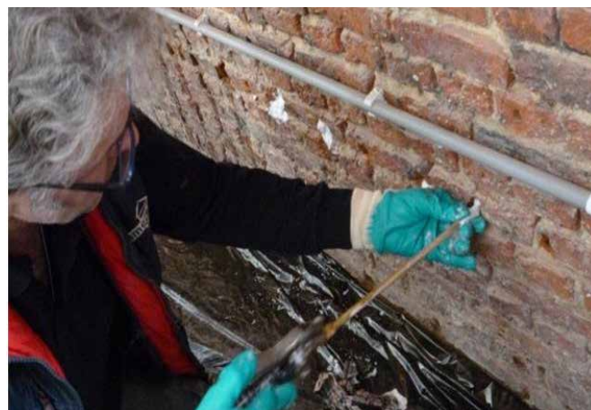
FIG. 3.6 Injection of a liquid product by means impregnation with a product in the form of a cream / Photo: B. Lubelli
