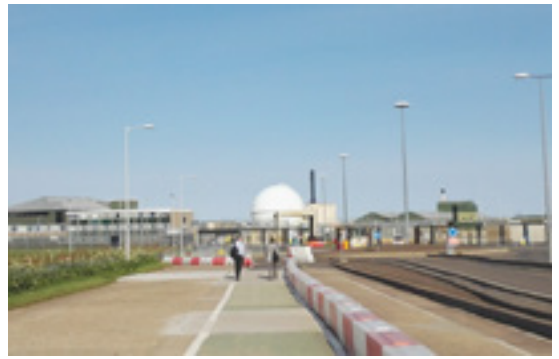
Dounreay Fast Reactor (Source: Photo taken by the researcher, Cara Mulholland)
