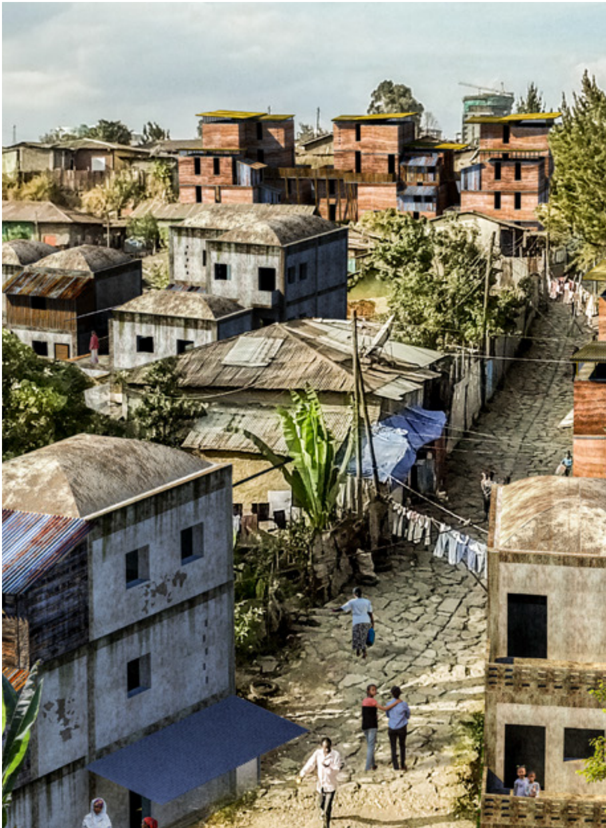
Project for the urban redevelopment of the Meneh neighbourhood, Addis Ababa (figure: Arianna Fornasiero and Paolo Turconi, 2017)
