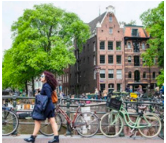
TOP: Historical photograph of Brouwersgracht 160 in Amsterdam BOTTOM: The same building today, identified from online street view images
