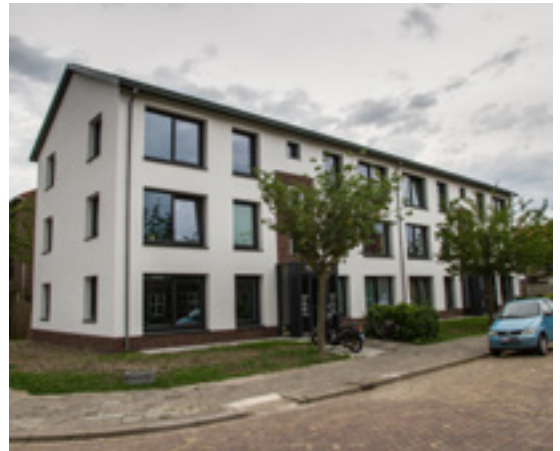
FIG. 5.2 2 nd Skin - Façade Refurbishment for Multifamily Social Housing. Picture: Marcel Bilow
