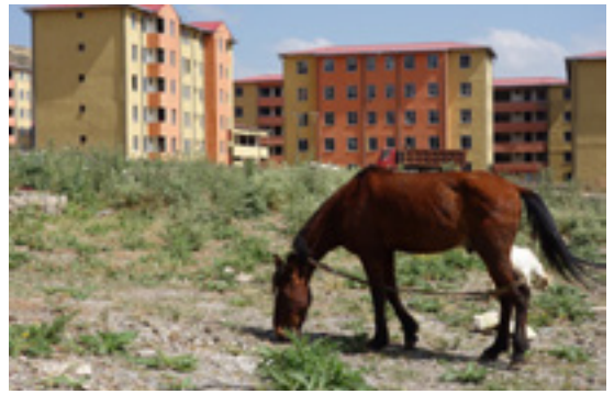
Yeka Abado condominium site. View of newly developed housing blocks, constructed on greenfields distant 20 Km from Addis Ababa city centre. November 2016 (photo: Nelson Mota)
