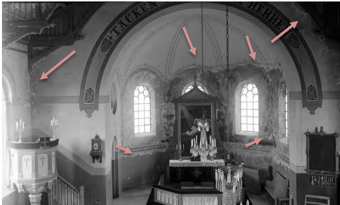
Figure 1: Extensive internal salt deterioration in 1920 in Smögen Church, designed by Adrian C. Peterson, built in 1905. The arrows indicate extensive salt damage. (Photographer Hanna Eggertz-Hegart 1920, kmb.raa.se, 2021-03-16).
