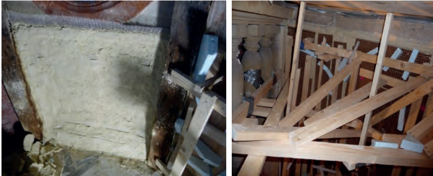
Figure 4: Test with (fibreglass) stucco mesh (left) and clamping of the poultice (right).
