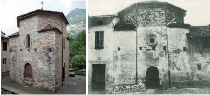
Figure 1: a) Current view of the Baptistery. (Photograph by A. Vattilana, courtesy of the Municipality of Riva San Vitale); b) The Baptistery before the restoration in the 1950s [4].
