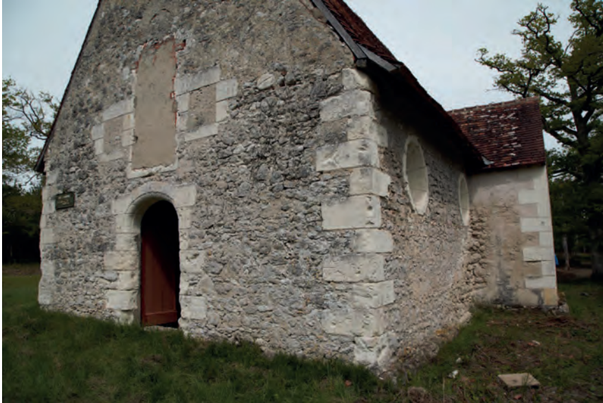
Figure 1: Photograph of the Chapel of Maurepas located in the Domaine National de Chambord, France.
