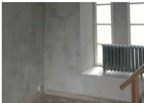
Figure 7: Lime plaster finish of NHL3.5.
