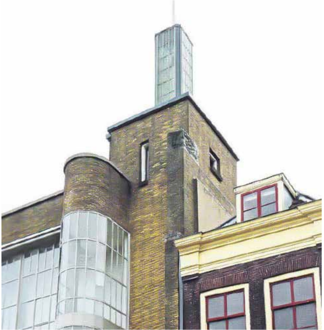
9. PHOTO OF THE CURRENT SITUATION OF THE VOORSTRAAT FACADE
