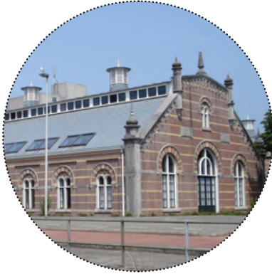
Pumping station building 1884-1888
