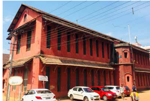
FIG. 8 19 th Century Administrative Office – Present DC Office Premises. Source: Author
