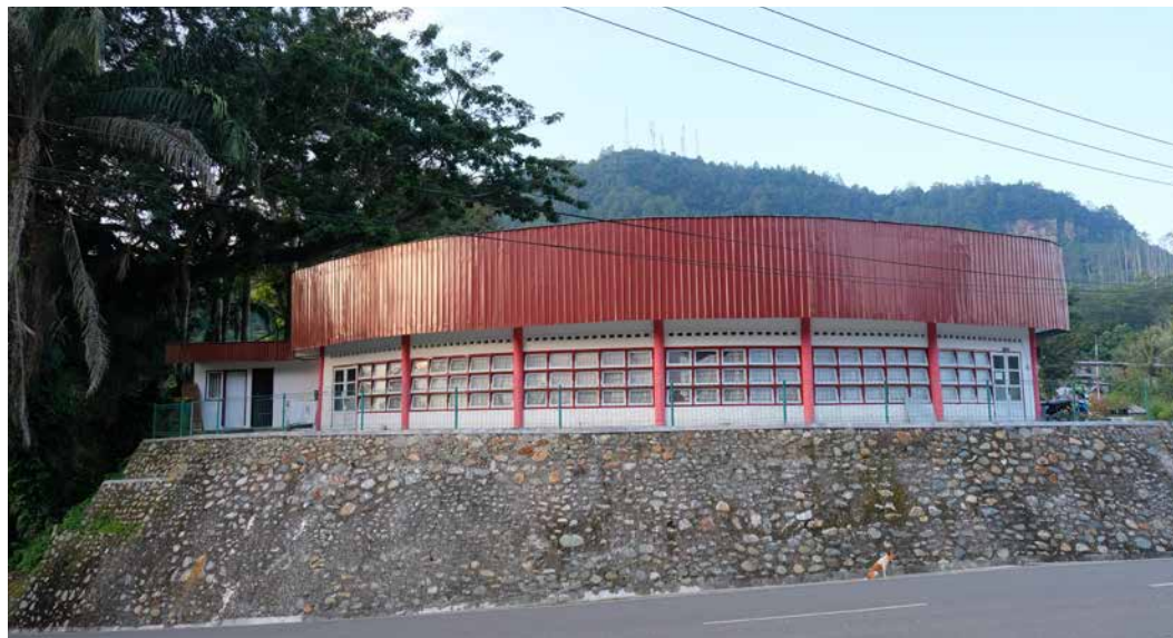
FIG. 6 Former Mining School. Source: author, 2019.
