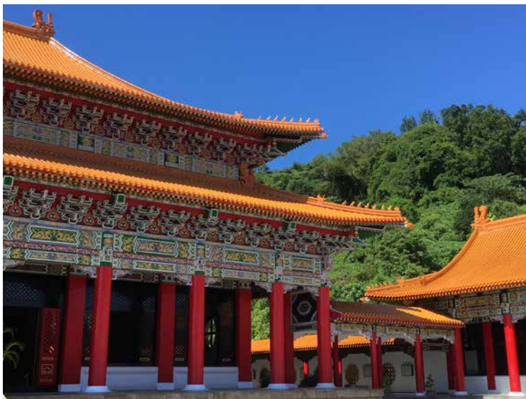
FIG. 3 Grand imperial yellow double-eaved roof decorated with auspicious animals—an architectural order exclusive to the Qing Emperors in Beijing, now also in Taipei. Source: author's own photo.
