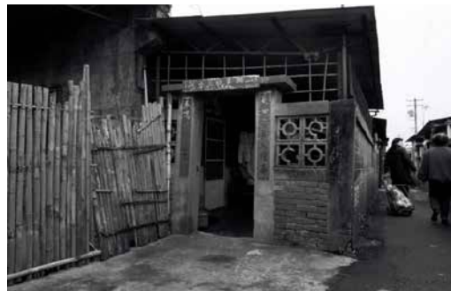
FIG. 9 Bamboo fence in Haiguang Fourth Village, Kaohsiung City. Source: Retrieved from http://blog.udn.com/wang32488/6367911
