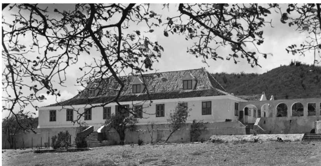
FIG. 14 Photo of the manor house of Landhuis San Juan in 1954. The arched aqueduct on the right directs the rainwater from the roofs to the regenbak (cisterns). Photographer: Van der Wal. Source: RCE.
