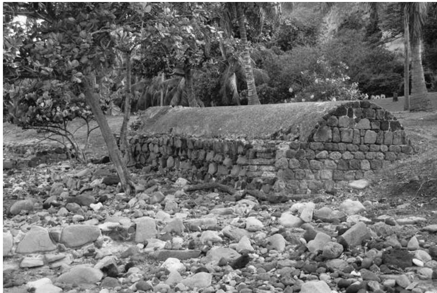
FIG. 17 Ruin of waterkelder/regenbak (cisterne) the benedenstad of Sint Eustatius. Relative high rainfall of 1200 mm (700-900 NL) turned Sint Eustatius into a strategic transshipment port in the Caribbean. Rainwater was 'harvested' and sold to cargoships. Today Bij gebrek aan adequate centrale watervoorziening worden bewoners in droge perioden geconfronteerd met drinkwater tekorten. Photographer: Saskia de Kock. Source: RCE.
