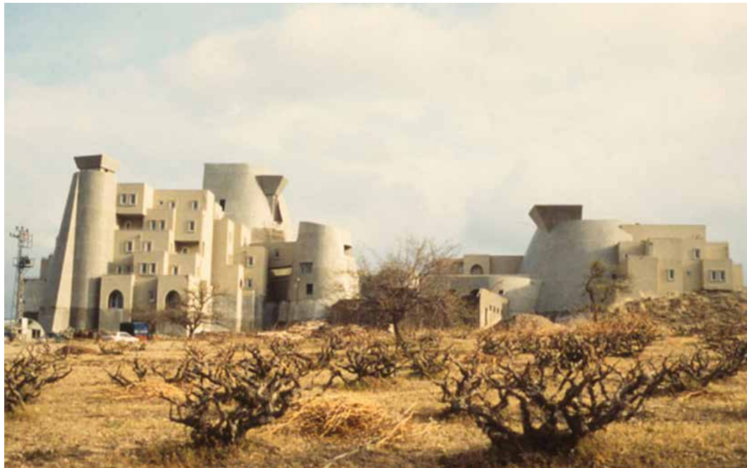
FIG. 5 The Peritower Hotel. Source: https://archnet.org/sites/1319/media_contents/21924
