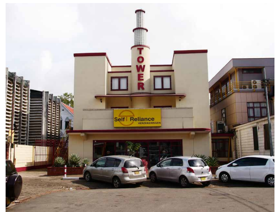
FIG. 2.18 Parkeren op de voetpaden Parking on sidewalks is still accepted
