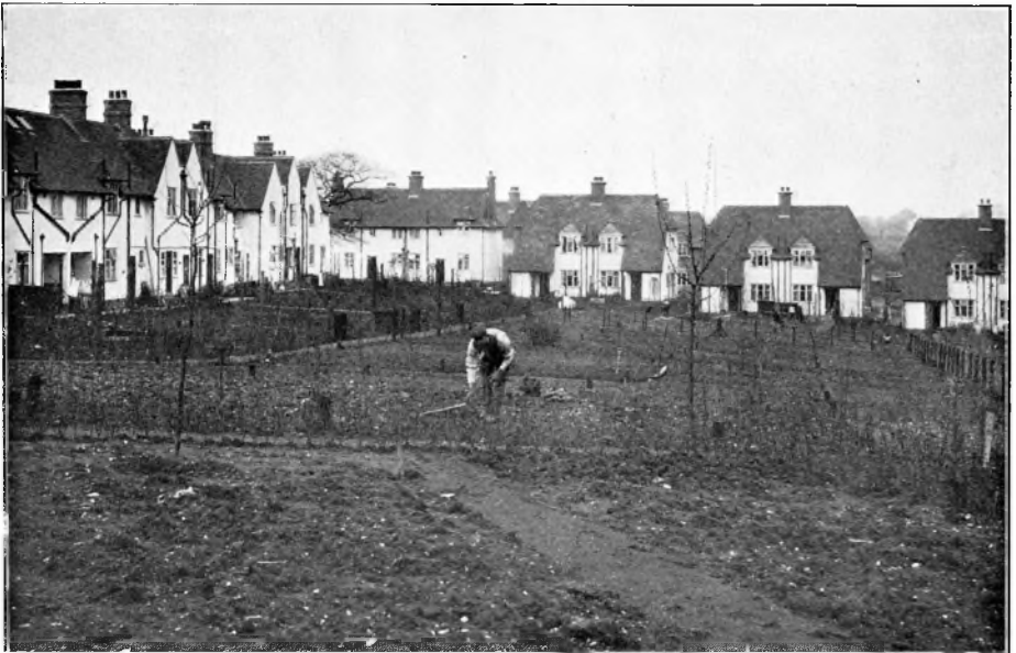
BACK VIEW, SHOWING THE AMOUNT OF OPEN SPACE, WITH 12 HOUSES TO THE ACRE NET, OR ABOUT 10 GROSS, AS IN SCHEME IIa.
