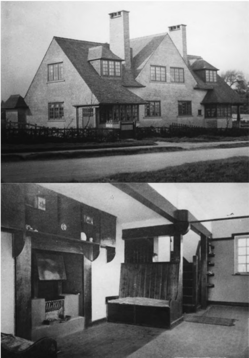
Figure 7 Cottages at Starbeck, Harrogate, Barry Parker and Raymond Unwin, 1903, developed from the scheme for 'Cottages near a town' exhibited at The Northern Artworkers' Guild in Manchester. The fitted furniture and inglenook fireplace from 'An Artizan's Living Room' has become a reality. (Parker Collection, First Garden City Heritage Museum, Letchworth.)
