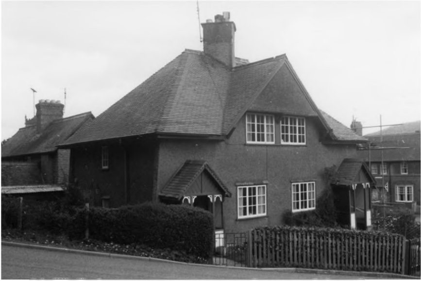
Figure 6 Cottages in Cunnery Road, Church Stretton, Barry Parker and Raymond Unwin, c.1900-01. This unassuming semi-detached pair became a prototype for housing at New Earswick and Letchworth. (Author's photograph.)
