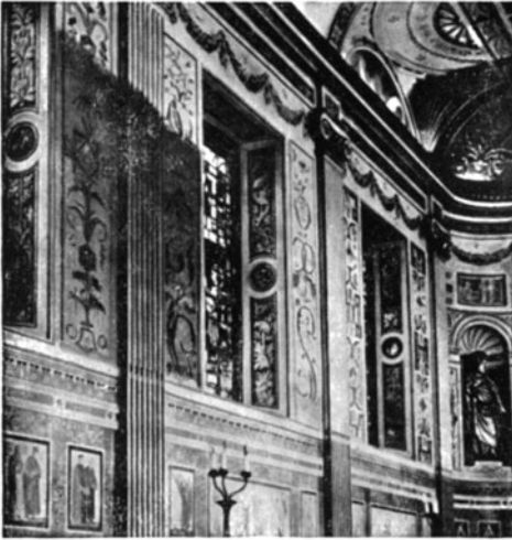
A pre-restoration view of the sombre shade of part of the interior wall, in remarkable contrast with cleaned areas.
