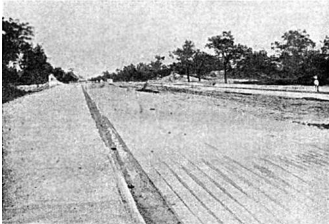
THE BUILDING OF GARY. Completing the Roadways.
