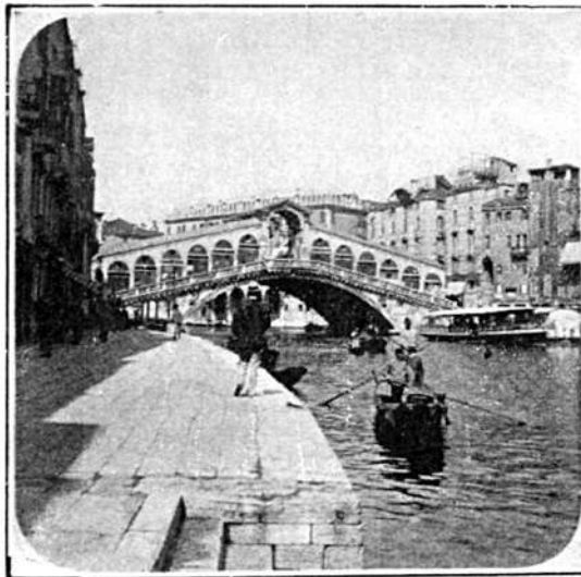
THE WATER HIGHWAY. Its Widest Utilisation at Venice.
