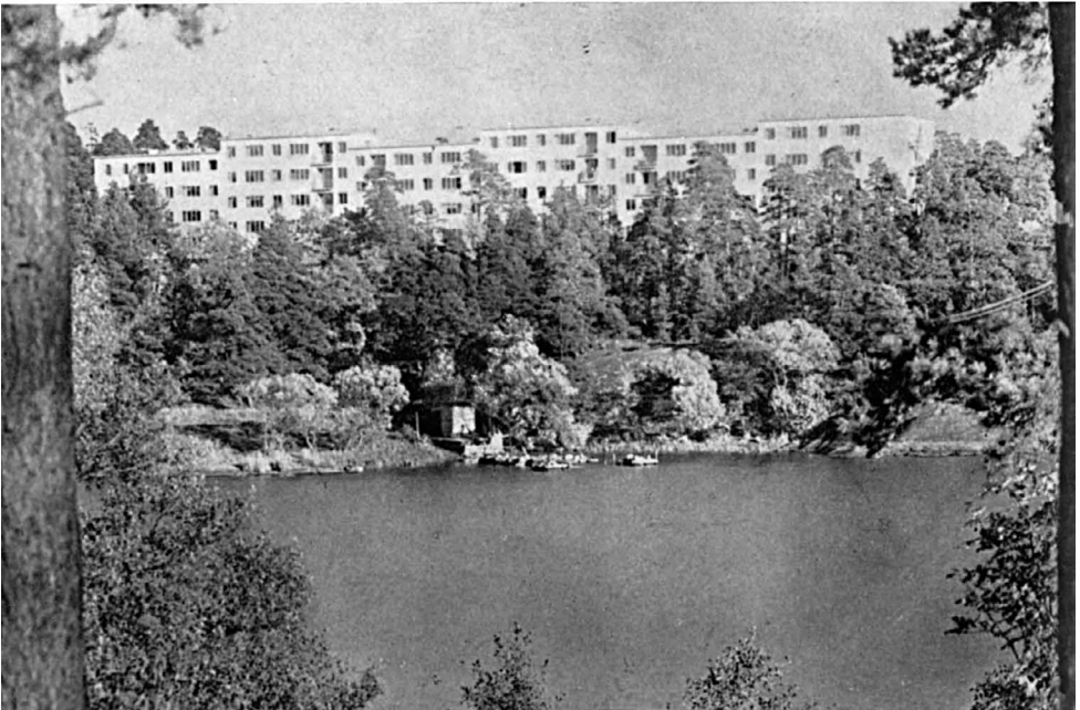
An H.S.B. block for workmen. The "stepped" roof was economical, enabling entrances to be made to flats from the half landings of the internal staircases
