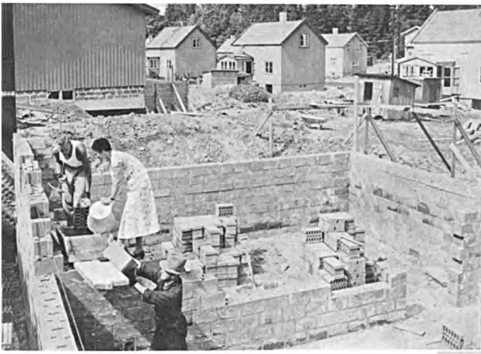
(a) Work on the foundations
