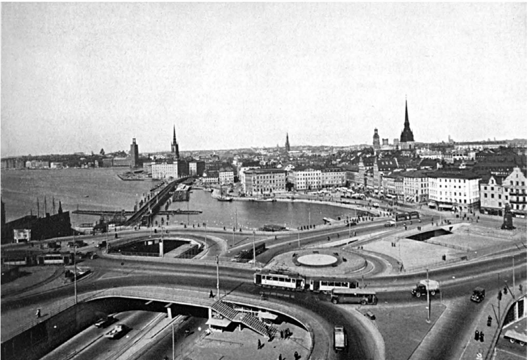
The new road linking the old town to the mainland. The spiral viaducts enable traffic to flow smoothly in any direction without impediment
