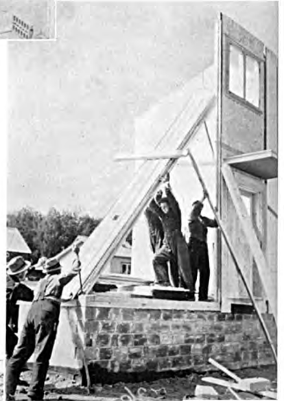
(b) Raising the timber walls into position
