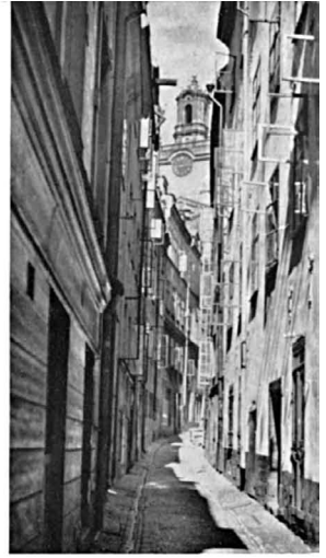
A typical street. The ground floors are mainly condemned as living quarters
