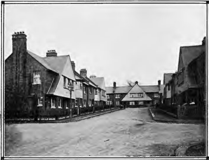
SOTTERDOWN ESTATE. — CLABURN ROAD FROM SOUTH WEST
