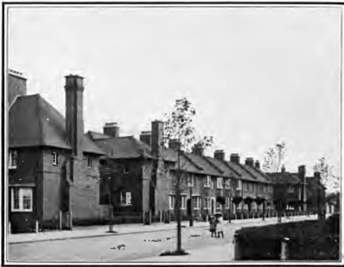
WHITE HART LANE ESTATE. — (AWLFIELD AVENUE)
