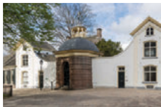
6. Dome as main entrance 2017
