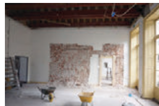
3. Ceiling in transformation
