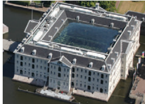
2. Aerial view of the building with the glass dome
