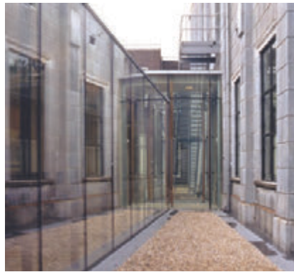
2. Henket extension (l) and old building (r)
