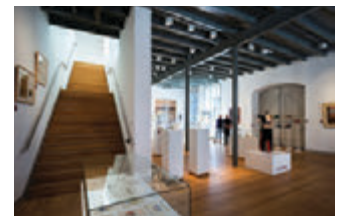
4. Ceiling with added steel structure
