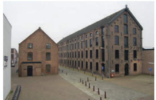
3. Entrance before the transformation
