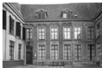
7. Original building entrance
