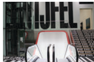
3. Escalator tube which connects the rooms upstairs and the basement
