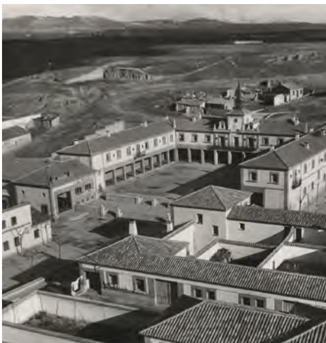
D.G.R.D. Reconstruction de Las Rozas: plan, aerial view of the ruins, aerial view of the new Plaza Mayor, aerial view of the new rural units. © AGA.
