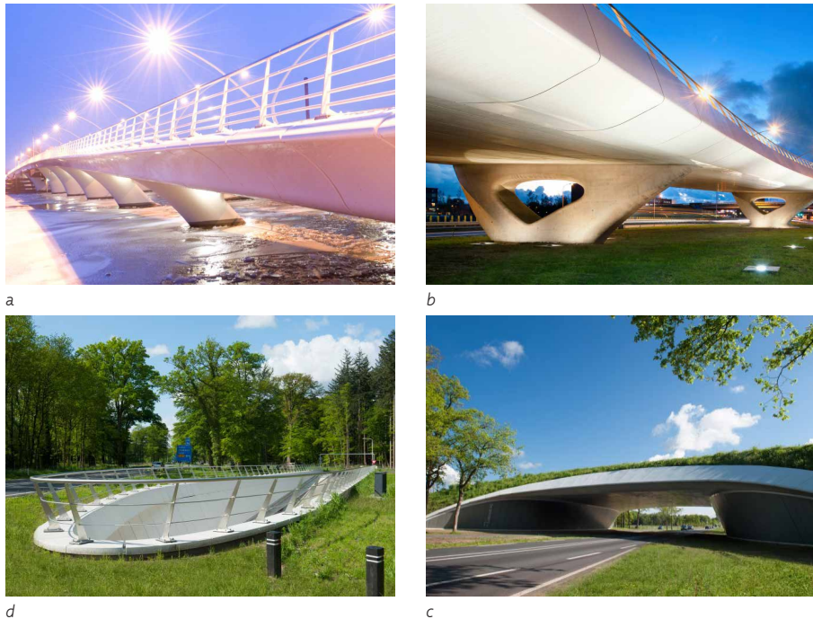
FIGURE 4.9 Some projects in the Netherlands with FRP edge elements, clockwise from top left: Edge elements on the Juliana Bridge in Zaanstad (a); The fly-over Waarderpolder in Haarlem (b); The wildlife crossing and tunnel in Rijssen-Wierden (c, d). Royal HaskoningDHV, Joris Smits et al., (2007, 2013, 2013). Photo's Jane van Raaphorst.
