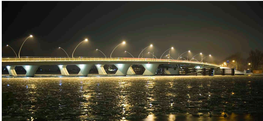
FIGURE 2.9 The opening part of the Juliana Bridge is in harmony with the approach spans. Royal HaskoningDHV, Joris Smits et al. (2009). Photo by Jane van Raaphorst 2010.
