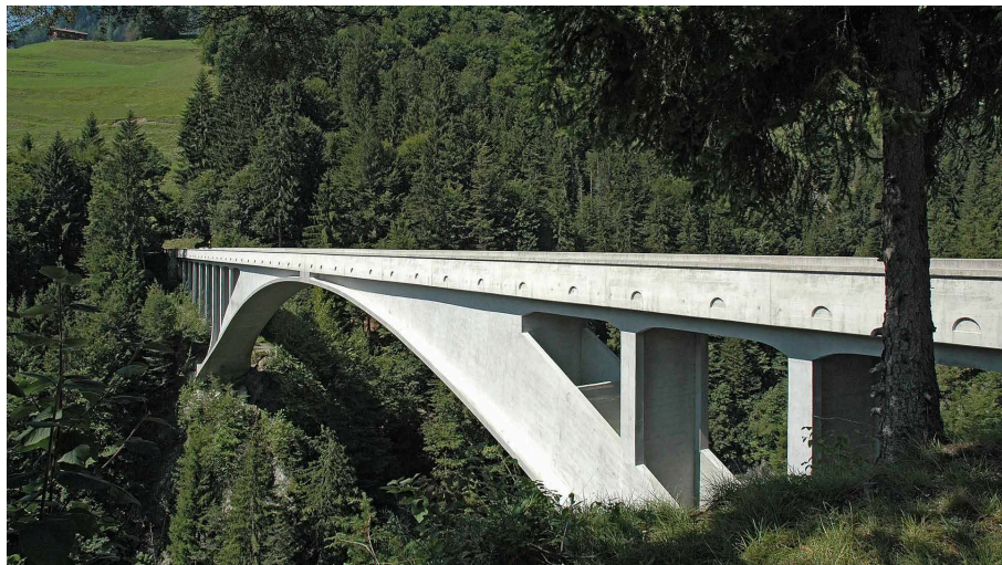
FIGURE 1.5 Salginatobelbrücke in Zwisserland (Robert Maillart, 1872- 1940). Photo from https://grandtour.myswitzerland.com . visited on 25/02/2019.
