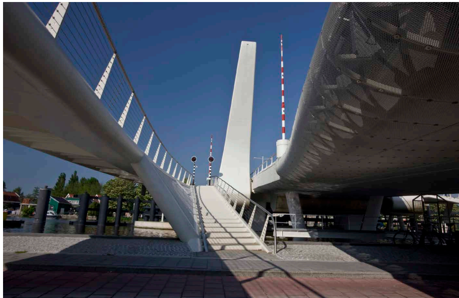
FIGURE 2.6 The Prins Bernhard Bridge, a multi-layered bridge with access to the quays. Royal HaskoningDHV, Syb van Breda and Joris Smits et al. (2007). Photo by Jan van Oevelen 2008.
