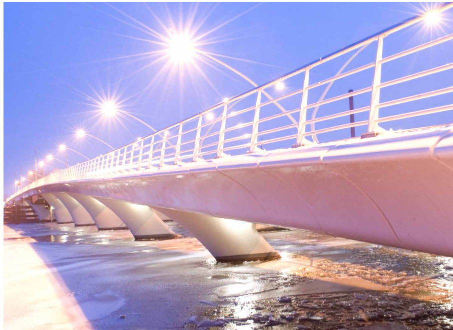
FIGURE 2.13 The horizontal manifestation of the deck with set-back of the piers puts the emphasis on the larger scale and blends into the landscape. Royal HaskoningDHV, Joris Smits et al. (2013). Photo by Jane van Raaphorst 2010.
