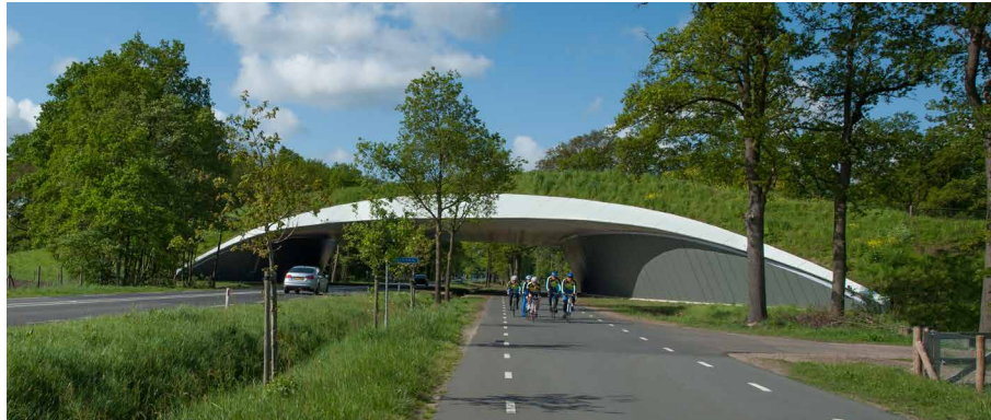
FIGURE 2.20 'Lifting the carpet' leaves a slit-like opening underneath the green structure. The low parts of the slit are filled with solid abutments with a set back from the edge. They are materialised in a dark grey colour in order to blend with the ground rather than with the crescent edge. This results in the impression of one long continuous edge. Royal HaskoningDHV, Joris Smits et al. (2014). Photo by Jane van Raaphorst 2014.
