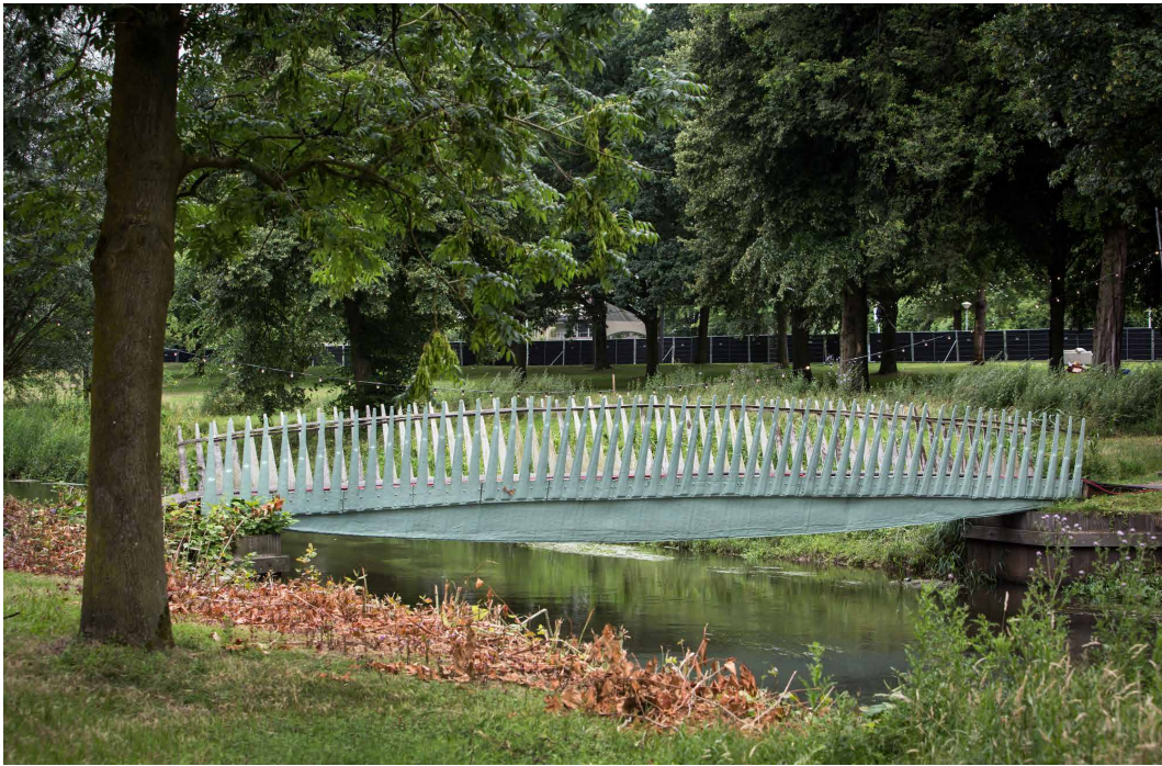
FIGURE 5.1 The bio-composite footbridge, 18 months after the installation across the river Dommel. R. Blok, J. Smits et al., Eindhoven University of Technology & Delft University of Technology, (2017). Photo by Heijmans (2018).
