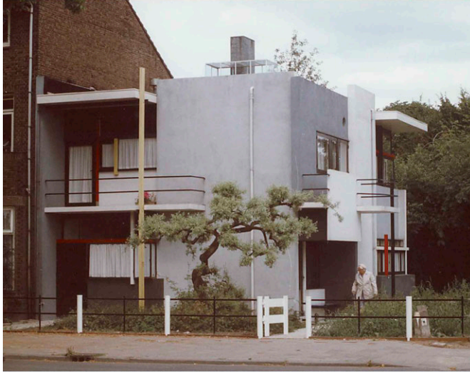
FIG. 2.6 The house in the early 1980s, after the second treatment of the exterior
