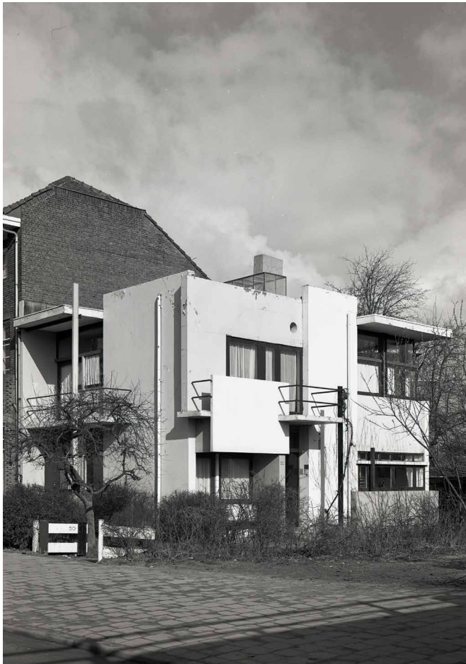
FIG. 1.1 In the beginning of the 1970s the state of repair of the Schröder House left a lot to be desired
