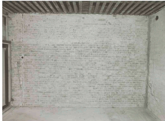
FIG. 3.6 Bare brick wall and stripped ceiling
