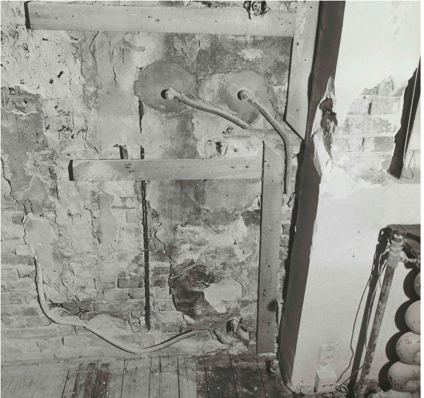
FIG. 3.1 The dismantling of wall, floors and ceiling yielded a lot of information about pipes, connection points and the attachment of furniture
