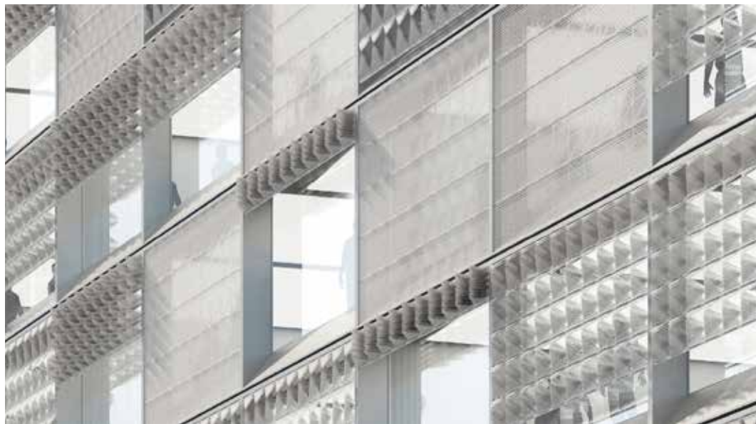
FIG. 18 Folded and cut spacer textile for exterior sun protection
