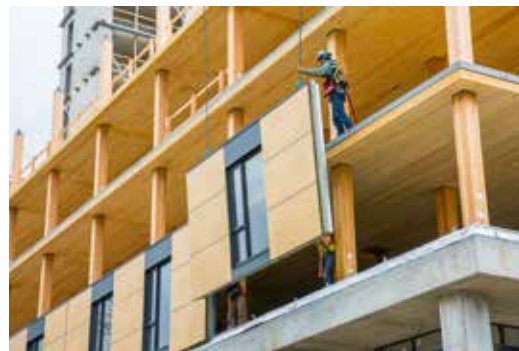
FIG. 12 Brock Commons fully prefabricated envelope installation phase (source: www.naturallywood.com )
