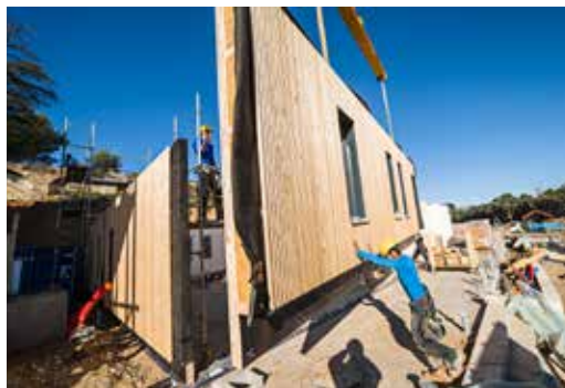
FIG. 11 Facade installation process for the Nexity Ywood «L'Ensoleillée II» building in Aix-en-Provence (source: © Nexity, Yann Bouvier)
