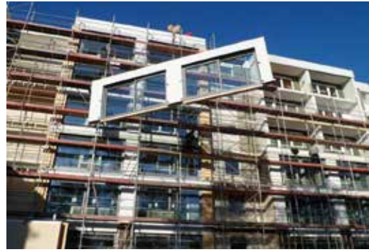
FIG. 2 TES EnergyFacade project – panel installation (source: Gump & Maier)
