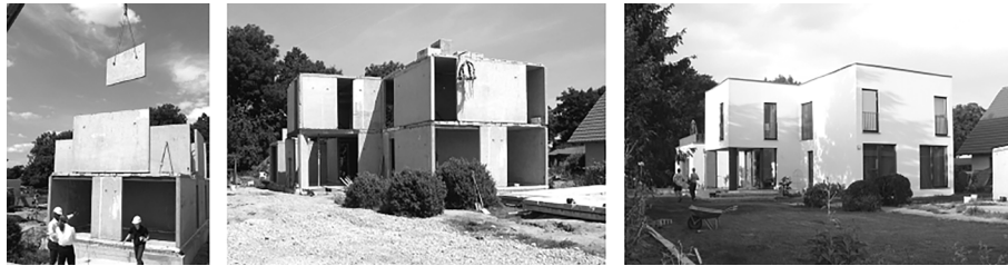
FIGURE 5.2 Pilot house in Mehrow near Berlin (Architecture bureau CONCLUS) (Claus, 2007).
