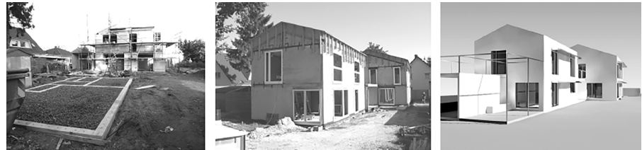
FIGURE 5.3 Pilot house in Schildow near Berlin (Architecture bureau CONCLUS) (Claus, 2007).
