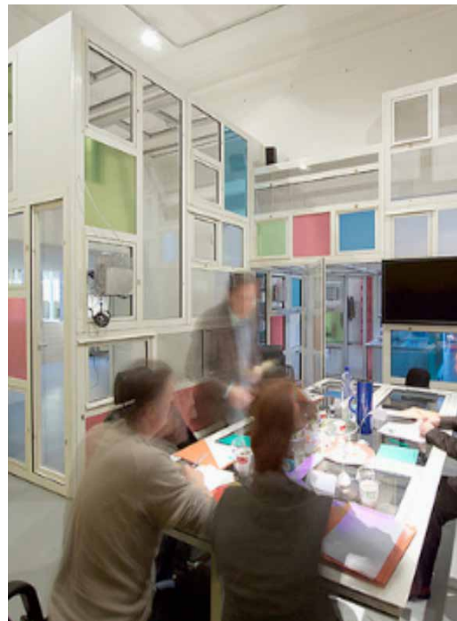
FIGURE 5.6 PVC office partition ( www.superuse-studio.com ).
