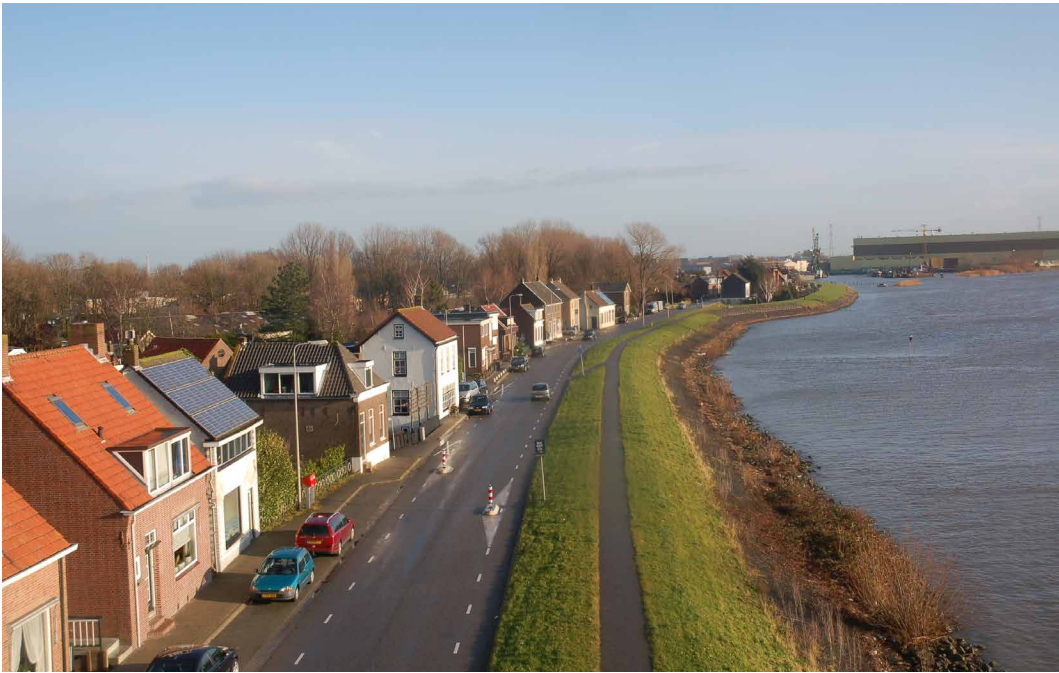
FIGURE 5.5 Photo of the Sliedrecht levee along the Merwede, incidental built constructions and trees on the riverside have been removed for dike reinforcements
