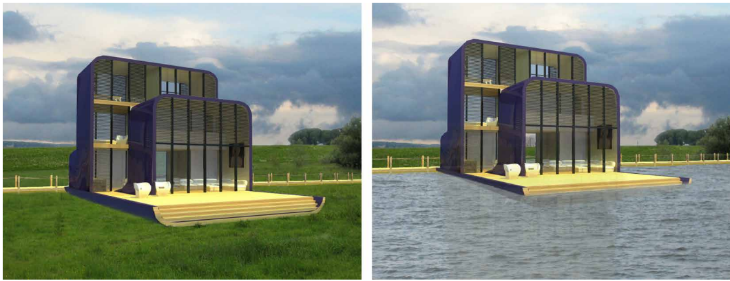
FIGURE 2.4 Design for a lightweight composite amphibious house for retention areas.
