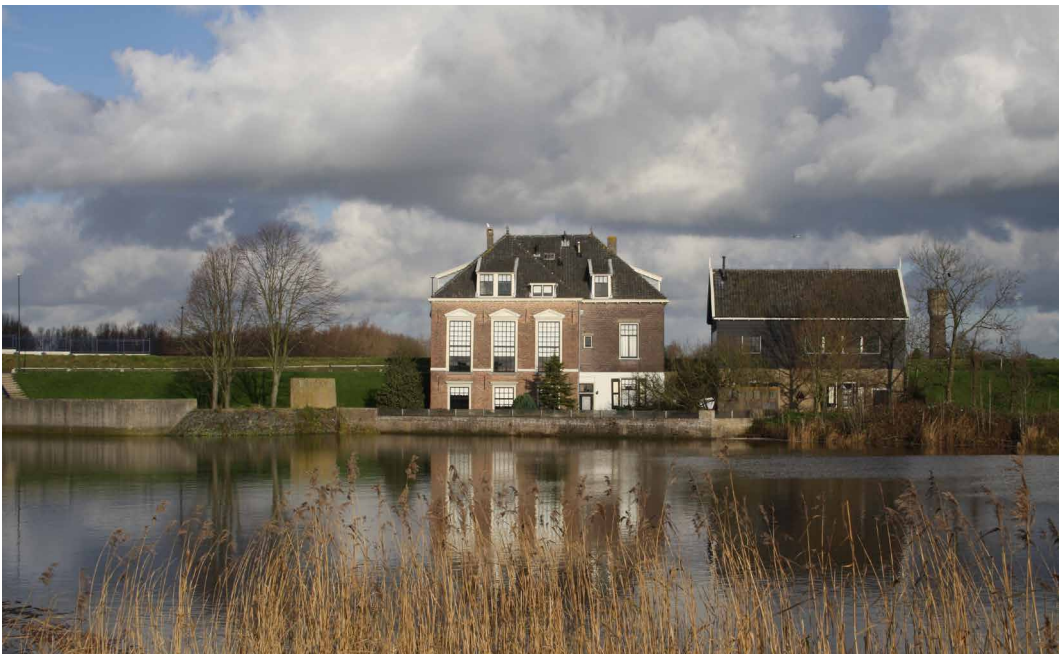
FIGURE 5.6 Photo of the monumental house of the water board on the polder site of the river Lek dike, within the Kinderdijk UNESCO area
