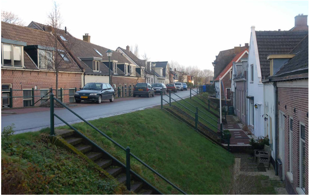
FIGURE 5.7 Photo of a previous levee elevation on a two-sided built levee along the river Lek near Everdingen
