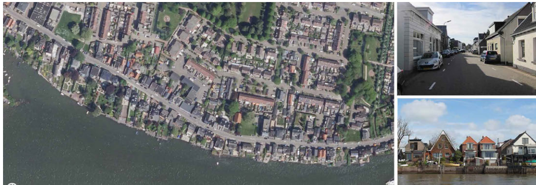
FIGURE 8.11 Aerial photo of the Rivierdijk in Sliedrecht (source: PDOK). On the right, a photo of the built dike from the road (centre of the dike) and from the river.
