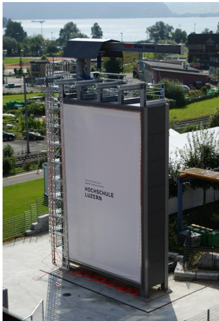
▶ Fig. 1: EN 13830 test facility at Lucerne University of Applied Science and Arts, Horw Switzerland
