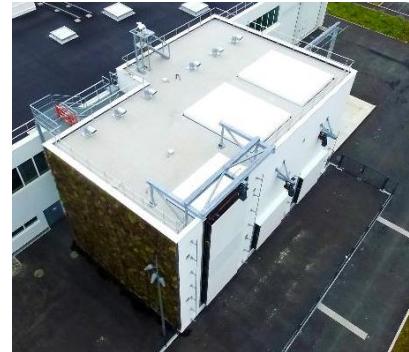
► Fig. 1: Full view of test facility
