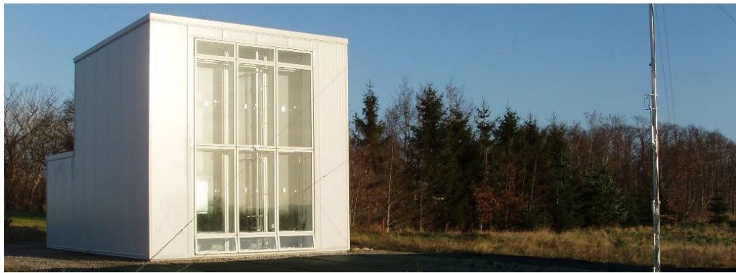
Figure 2 - The Cube, outdoor test facility with DSFV.
