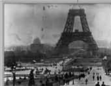
1889 Eiffel Tower (Eiffel)
