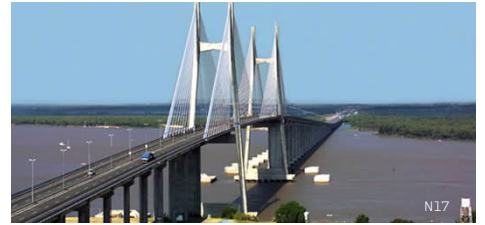
2003- Construction of Rosario-Victoria 4 Km-long Bridge (RN174) ▶
