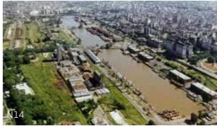
Puerto Madero before works
