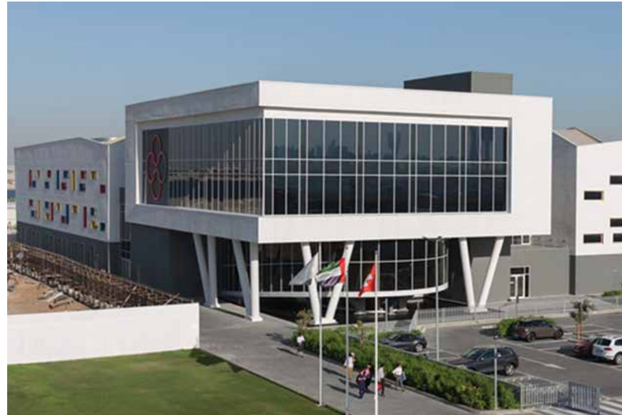
Main view on the electrochromic facade, Swiss International School in Dubai (WME Consultants, UAE)
