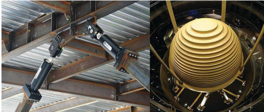
**FIGURE 1.1** Viscous dampers integrated in a braced frame system (left) and a tuned mass damper hanging from the Taipei 101 building's roof (right). Sources: *engineeringfeed.com* and *civil-engg-world.blogspot.nl*, respectively.
