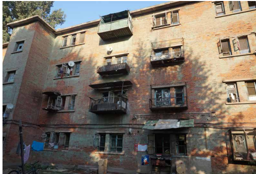
FIGURE 3.4 The external dwelling condition of a danwei community Source: Authors
