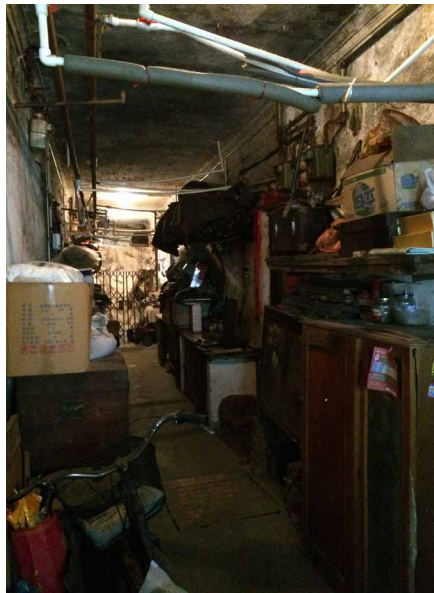
FIGURE 3.1 The internal dwelling condition of a danwei community Source: authors
