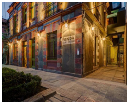
Figure 7: Images of the Havre 69 project at Mexico City. The picture shows the new relations with the urban tissue, the pedestrian life and mixed uses generated. Source: Metalocus. Available at: http://www.metalocus.es/es/noticias/hablando-con-la-ciudad-havre-69-por-at103-arquitectos
