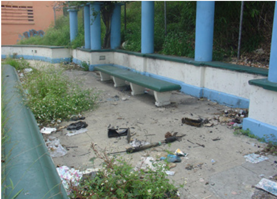
Figure 3: San Martin Plaza, Caracas, Venezuela. Degradation, uncleanness and mortification: an ordinary reality of many public spaces. Source: Angel Rincon. Available at: https://www.flickr.com/photos/elegancia/5918052849/in/dateposted/
