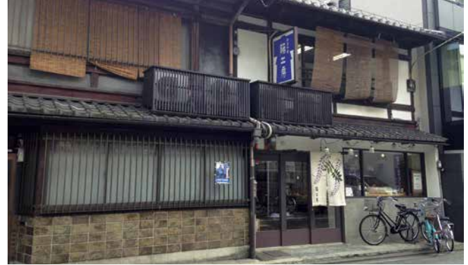
FIG. 22 Air-conditioning units covered behind specially designed wooden screens
