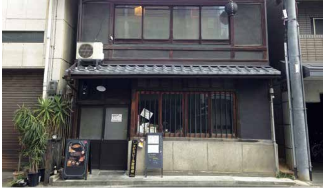
FIG. 21 Air-conditioning unit attached to the street façade of a machiya
