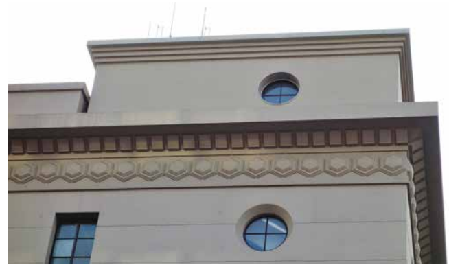
FIG. 16 Fortune Garden Kyoto, rooftop extension
