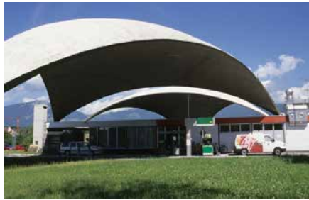
(a) Deitingen Service Station [24].
