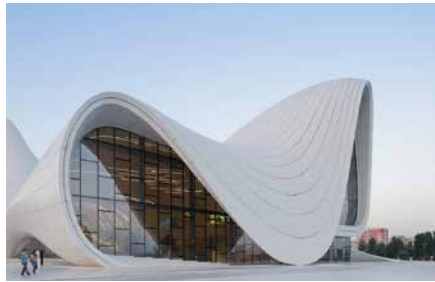
(a) Freeform roof.
