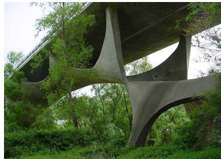
FIGURE 4.20 Figure 4.20: Basento Viaduct in Potenza, Italy, 1974 [108].
