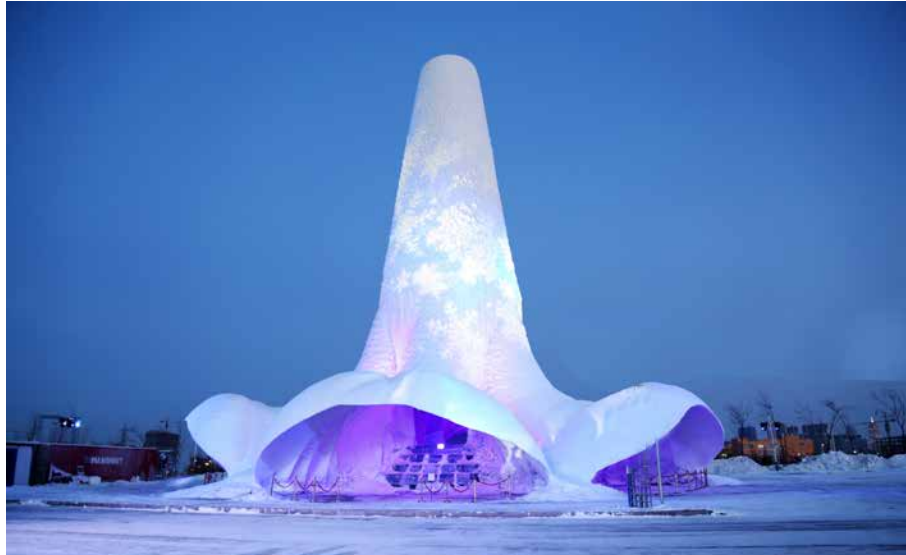
(b) The ice tower after construction (photo by Maple Village).
