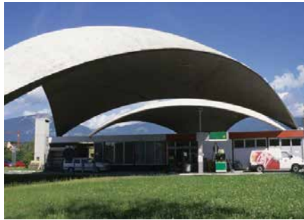
FIGURE 4.17 Deitingen Service Station, Switzerland, 1968 [104].
