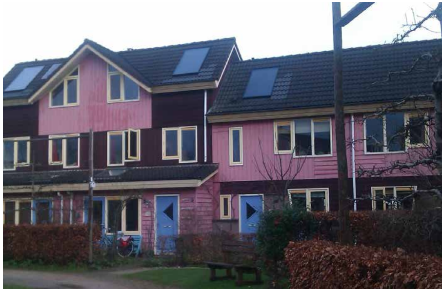
FIGURE 9.2 Bongerd (Zwolle): mixed typology; mixed use; mixed tenure but harmonised architecture. [picture: Tussen Ruimte, 2014]
