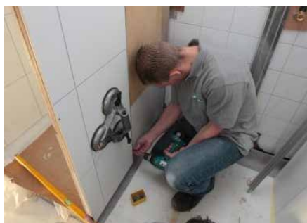
Renovatie badkamer/toilet (Bron: Faay)
