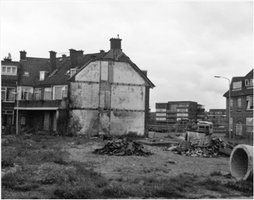
Figure 2.11 Duindorp: demolition due to social and structural problems
