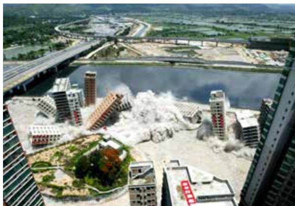
Figure 8.27 Demolition of Yunong Village Source: News Guangdong.
