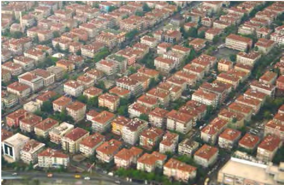
Figure 10 Gecekondu plots are merged to create larger properties suitable for five floor yap-sats.
