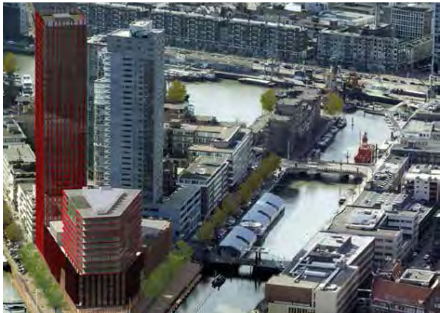
Figure 12 Towers of Wijnhaven Island in development.
