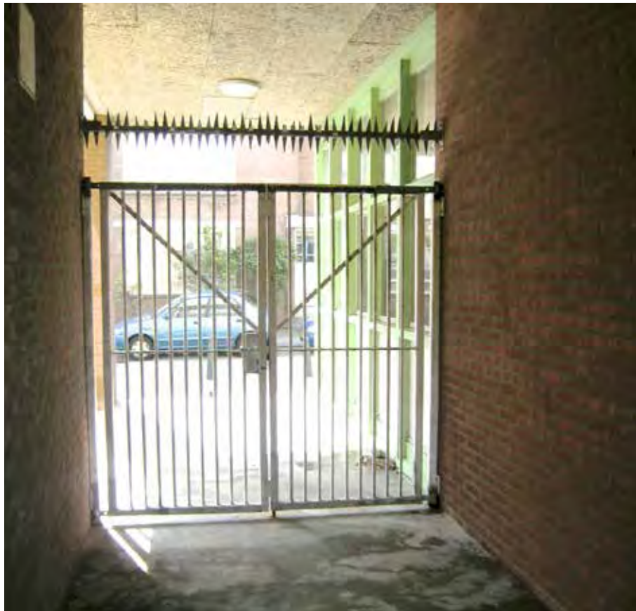
Figure 84 A locked courtyard gate in Oude Westen.
