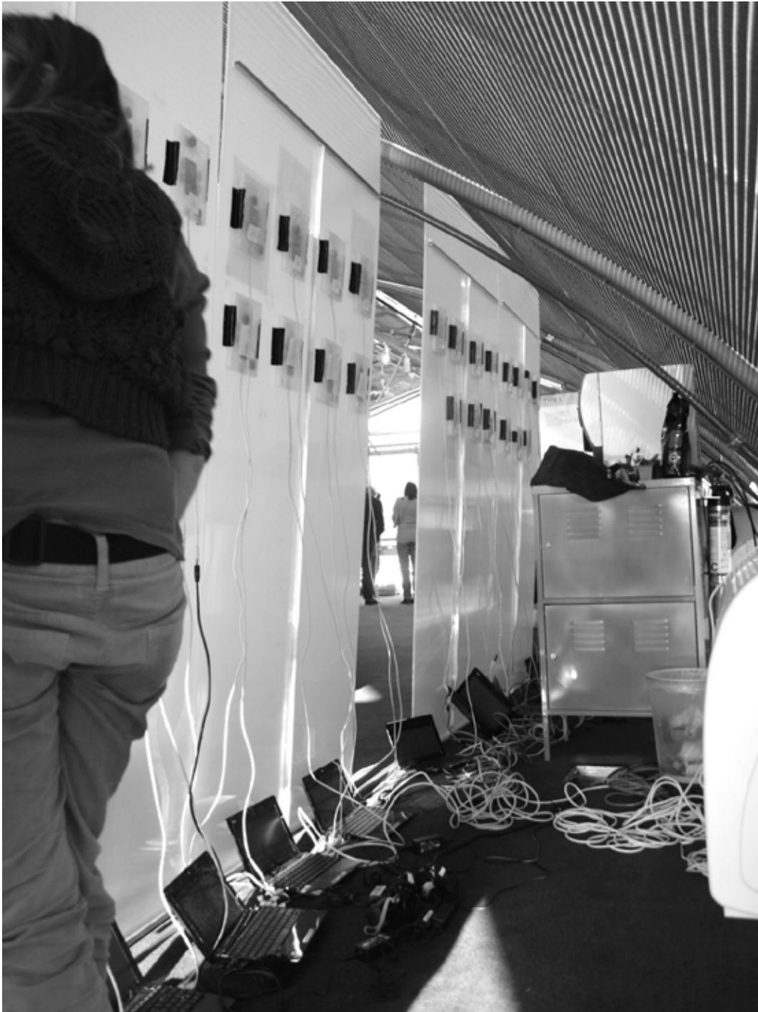
Figure 126 The technical equipment behind the voting station.
