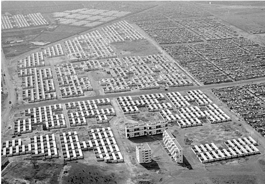
Figure 29 Aerial view of Casablanca's Carriere Centrale housing developments by the Group of Modern Moroccan Architects and Team 10 in 1952, adjacent to the oldest slum in North Africa.
