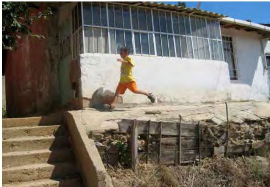
Figure 37 Various First Generation Gecekondu Homes in Gulensu.
