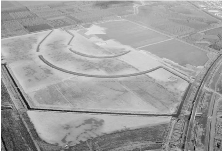
Figure 13 Homeruskwartier prepared for construction.
