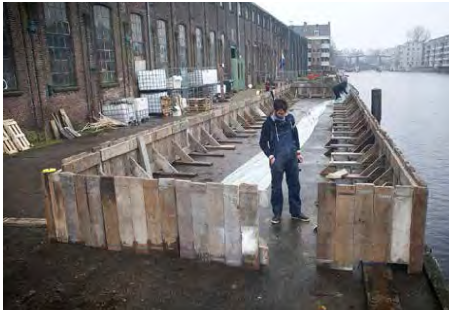
Figure 187 Tostifabriek under construction.
