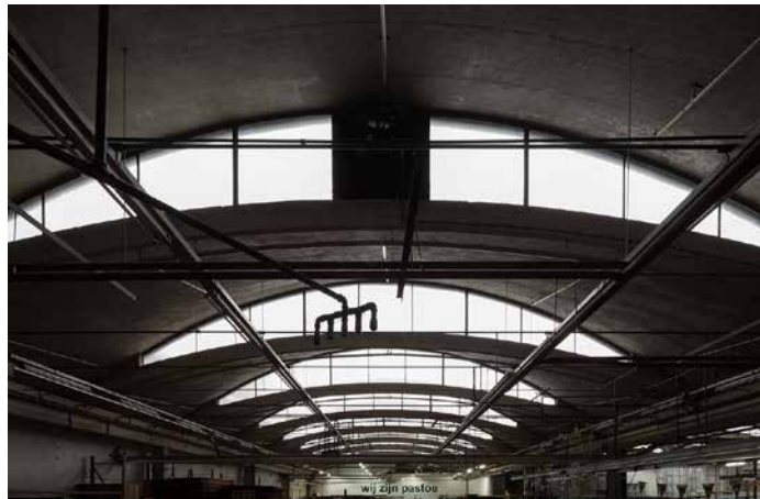
FIGURE 1.2 Conoid shells roofing the Pastoe workshop in Utrecht. Photo: Katja Eftting fotografie
