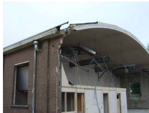
FIGURE 5.2 Demolishing building Q in 2012.
