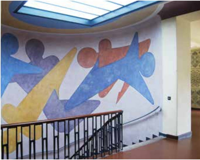
FIG. 3.32 Layers of time visible on the stairwell of the Van de Velde Building, Weimar, after the recent restoration of the Oskar Schlemmer mural leaving the remnants of the Schultze-Namburg period visible/ Marieke Kuipers
