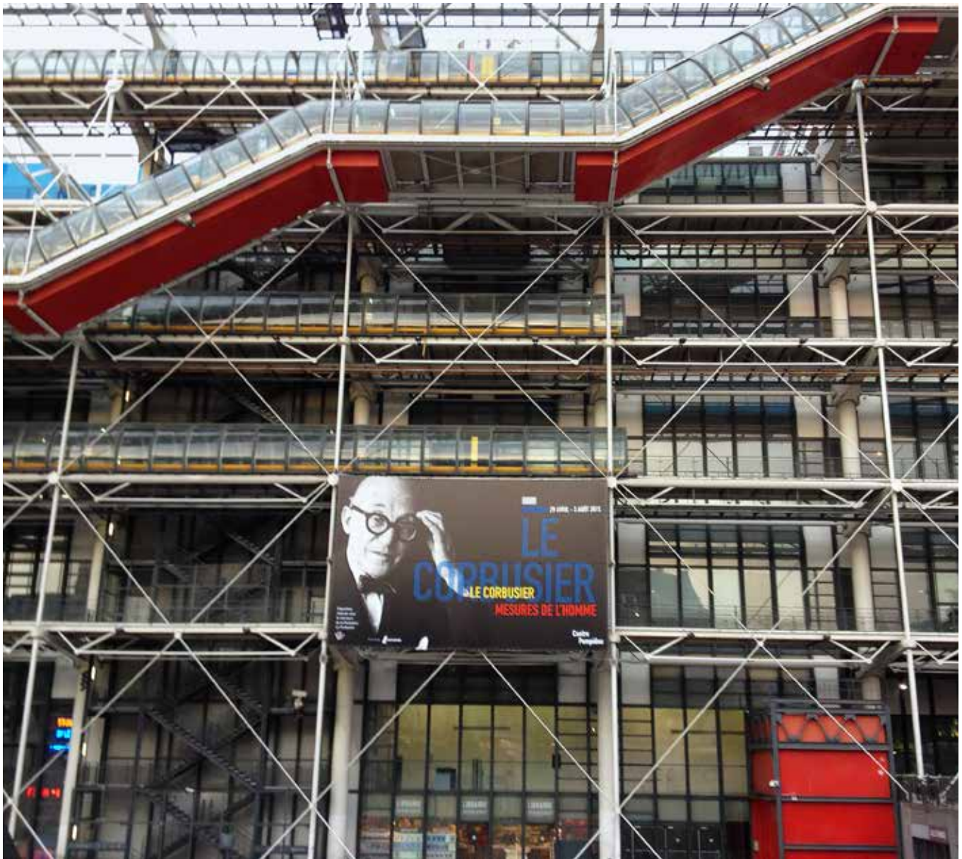
FIG. 3.19 The exterior escalators and tubes of the Centre Pompidou, Paris / Marieke Kuipers
