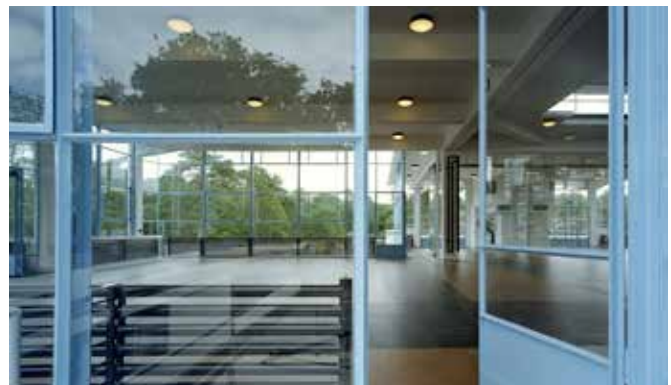
FIG. 2.17 Looking through the drawn glass into the main hall on the first floor, featuring tubular radiators, light fixtures and linoleum flooring that were remanufactured for the restoration / Jannes Linders
