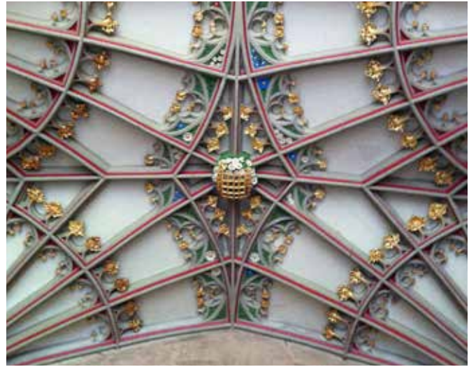
FIG. 3.33 Polychromatic articulation of the fan-vaulted ceiling, King's College Chapel, Cambridge / Marieke Kuipers
