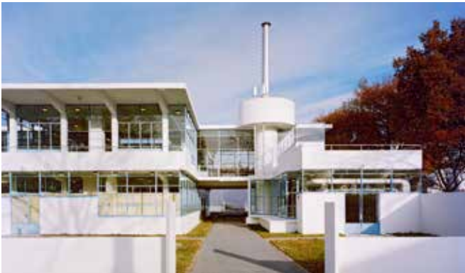
FIG. 2.15 The Main Building of Sanatorium 'Zonnestraal' after restoration in 2003 – a representation of the original idea and design intent, rather than original materials / Michel Kievits - Sybolt Voeten
