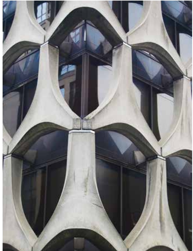
FIG. 3.28 The curtain wall composed of prefabricated wishbone-shaped elements (Ergon) of the former ALSK Bank, Brussels, designed by Marcel Lambrichts / Marieke Kuipers
