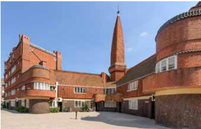
FIG. 2.2 Het Schip housing block in Amsterdam (Michel de Klerk, 1921) is an early example of a twentieth century building that was listed in 1974 already / Museum Het Schip .
