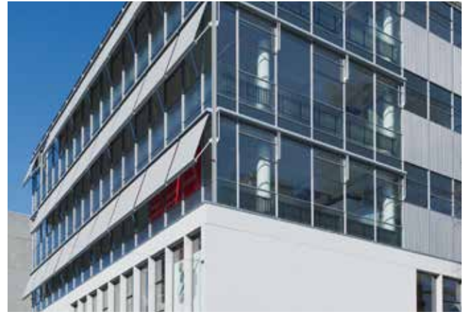
FIG. 5.17 The HUF Building restored in 2009; the newly installed awnings allowed for the use of clear insulated glazing units instead of sun reflective glass panels / Jannes Linders
