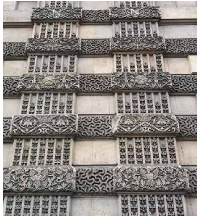
FIG. 3.18 The Seine façade of the Louvre, Paris, with sculptured animal decorations incorporated into the main structure / Marieke Kuipers
