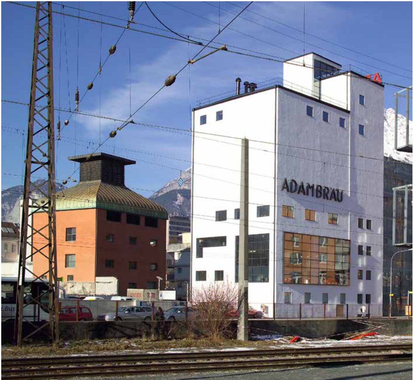
FIG. 2.18 The Adambräu Brewery in Innsbruck after restoration in 2008 / Christof Lackner
