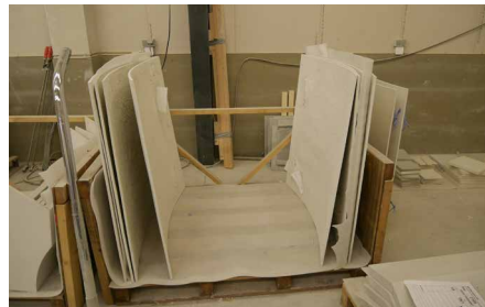
FIGURE 6.31 Finished cast panels for ring 1 and ring 2.
