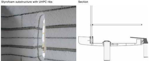
Styrofoam substructure with UHPC ribs
