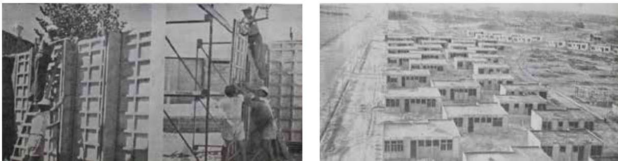
FIGURE 3 KALAD system. The left image shows the panels used for prefabrication in Narmak. The right image shows some houses constructed with this system in Narmak.
