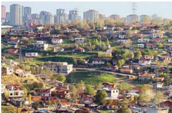
3 Redeveloped geoköndü areas - produced by the “share of construction” system since the late 1960s. These neighbourhoods are dominated by high density 4-6 storey apartment blocks, which have deteriorated over time, a high proportion of which are vulnerable to earthquake risk.
