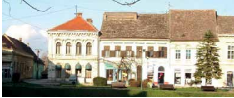
FIGURE 2 Pannonian type of housing with retail in the city centre of Sremska Mitrovica
