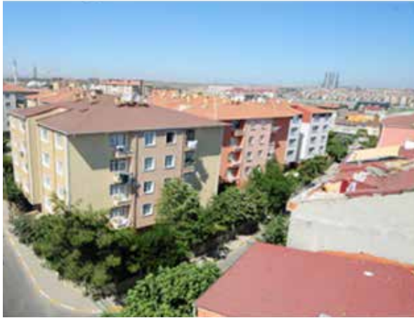
1 Barinkent Housing Estate: Apartment blocks before
