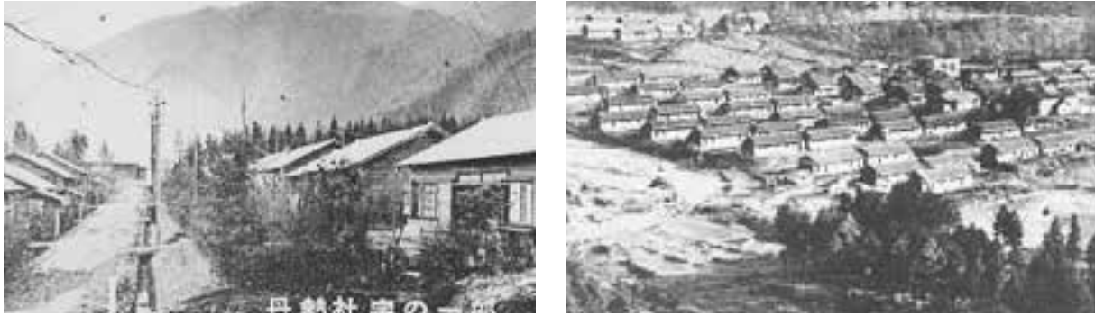
FIGURE 3 The Nikkō company houses. Tansei-Shataku (left) and Wanoshiro-Shataku (right).
