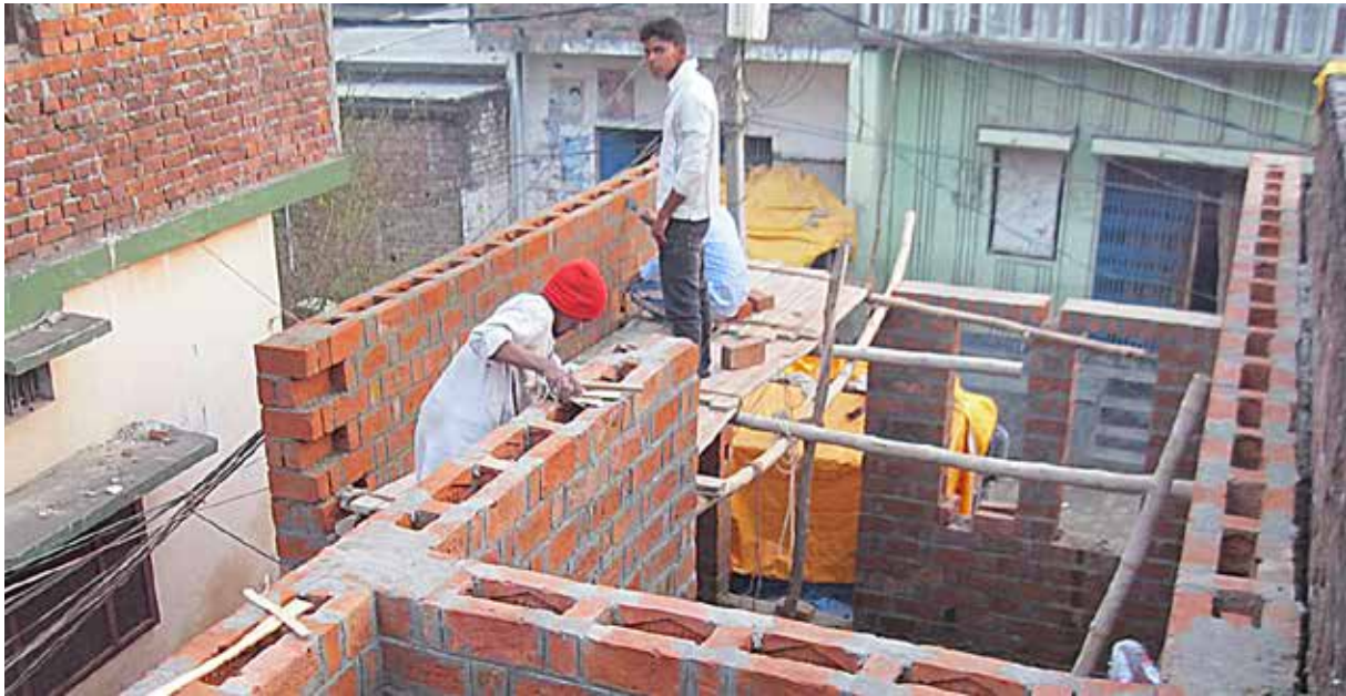
FIGURE 15 Construction of new homes designed with community inputs in Gorakhpur
