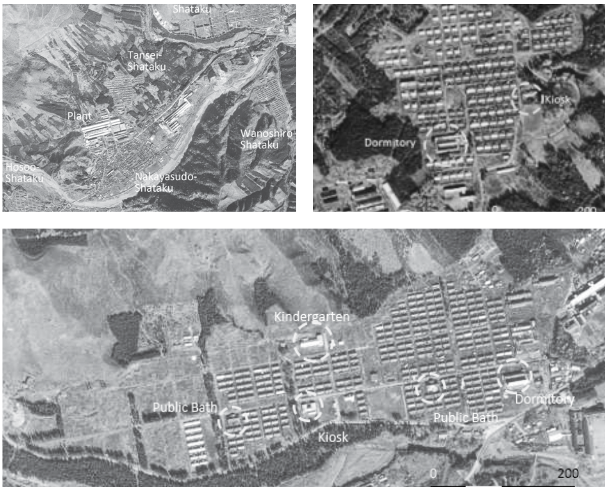
FIGURE 2 Nikkō Electric Copper Smelting Co.'s Industrial Village, captured in an aerial photo in 1963.
