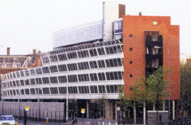
j. körmeling, 1989 kunsttoepassing / neon sign on top of mecanoos' hillekop housing, rotterdam 1989; j. coenen, na / netherlands architecture institute, rotterdam 1987 w. arets, w. van den bergh, jan van eyck-academie, maastricht 1989; s. soeters, woningbouw en kinderdag-verblijf \ housing and children day care, kinkerbuurt amsterdam 1982; r. uytenga, woningbouw \ housing droogbak, amsterdam 1990
