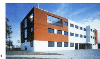
h. tupker, fnv horecabond kantoor | office, almere 1993
