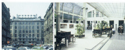
o. wagner, postsparkasse, in- en exterieur | interior and exterior, wenen | vienna 1912
