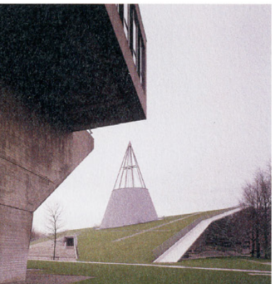
mecanoo, bibliotheek tu | university library, delft 1997 links de aula | at left, the 1967 auditorium
