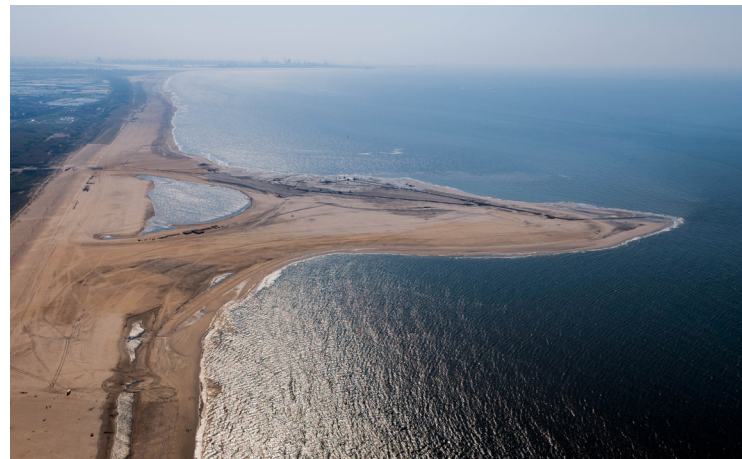
Figure 49. Sand Engine after completion in 2011. (Photo Courtesy Rijkswaterstaat/Joop van Houdt)
