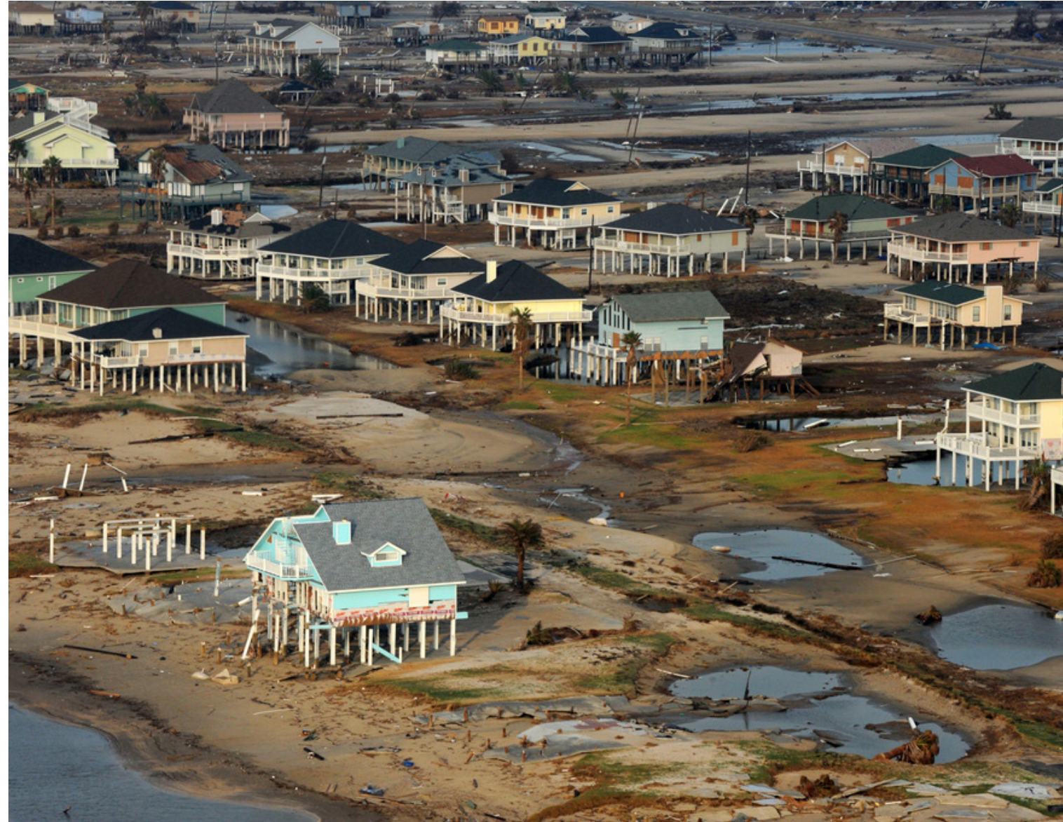
Figure 24. Destruction of homes on Bolivar Peninsula by Hurricane Ike. (Photo Courtesy Jocelyn Augustino, FEMA)
