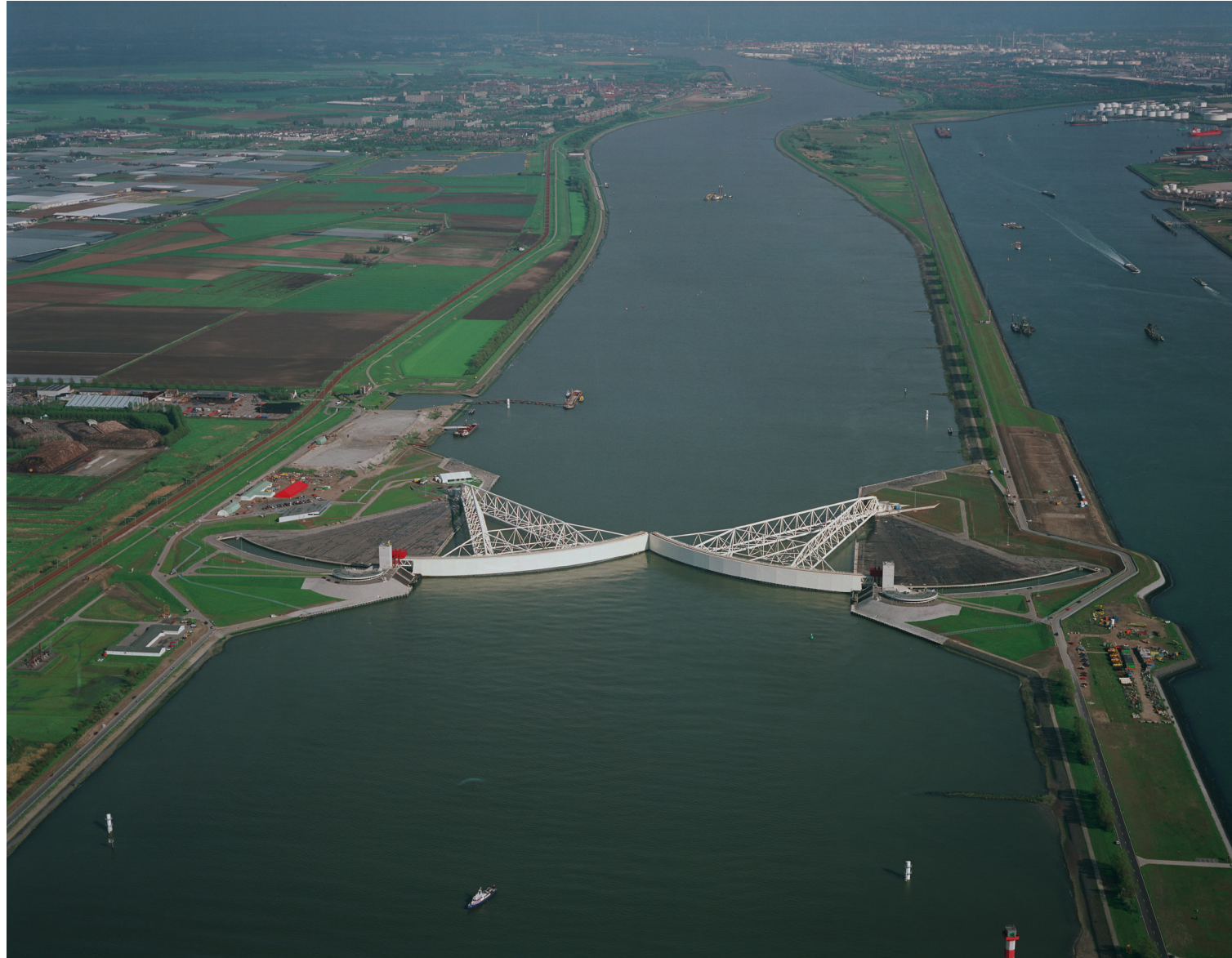
Figure 101. Annual test-closing of Maeslant Barrier in The Nieuwe Water- weg, shipping route to port of Rotterdam. (Photo Courtesy Rijkswaterstaat/Bart van Eyck)
