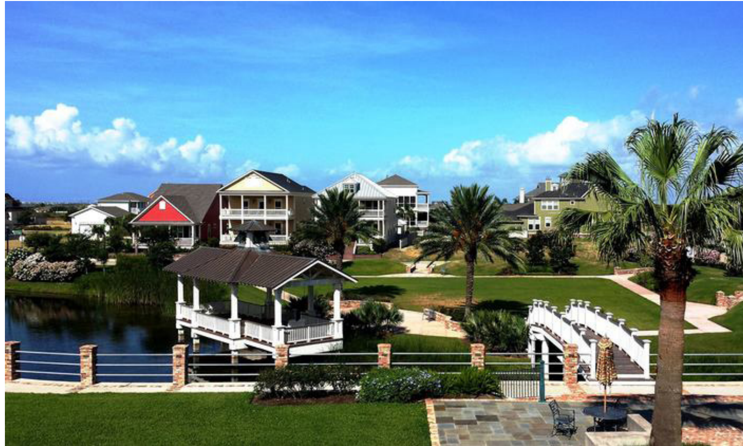
Figure 47. The Evia neighbor- hood on Galveston Island which survived Hurricane Ike with virtually no damage. (Photo Courtesy Sullivan Brothers)
