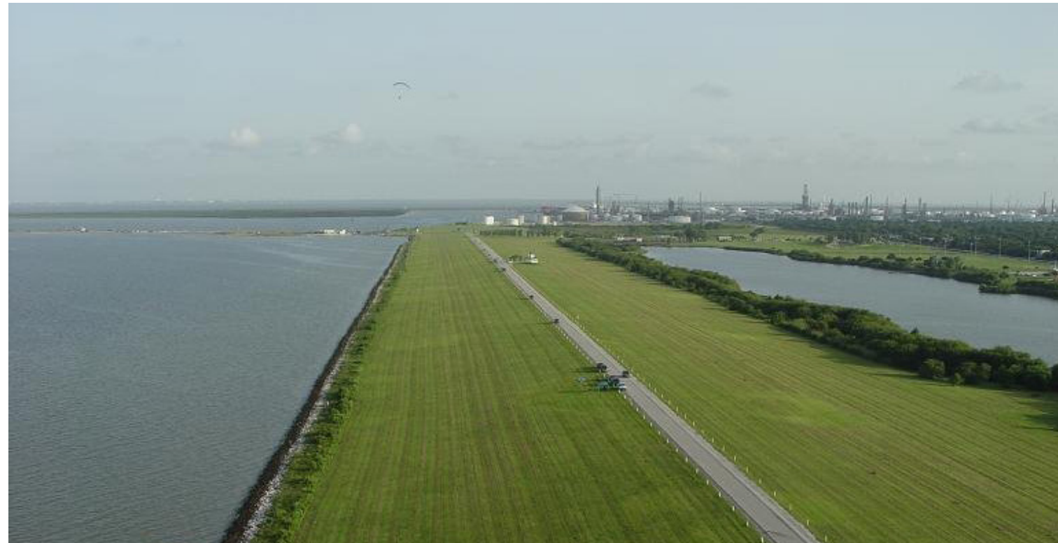
Figure 44. Texas City Levee. (Photo Courtesy KC10Chief)
