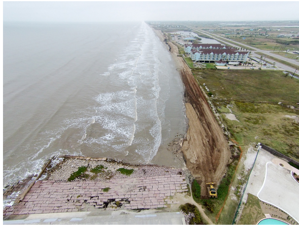
Figure 35. A bird's eye view on the Delanara-project at the west end of the Galveston Sea Wall. Beach nourishment is the product of a collaborative effort of the Park Board of Trustees, the City of Galveston, and the Texas General Land Office with the permission of three individual property owners. December 2014. (Photo courtesy Dustin Henry, Planning Department City of Galveston)
