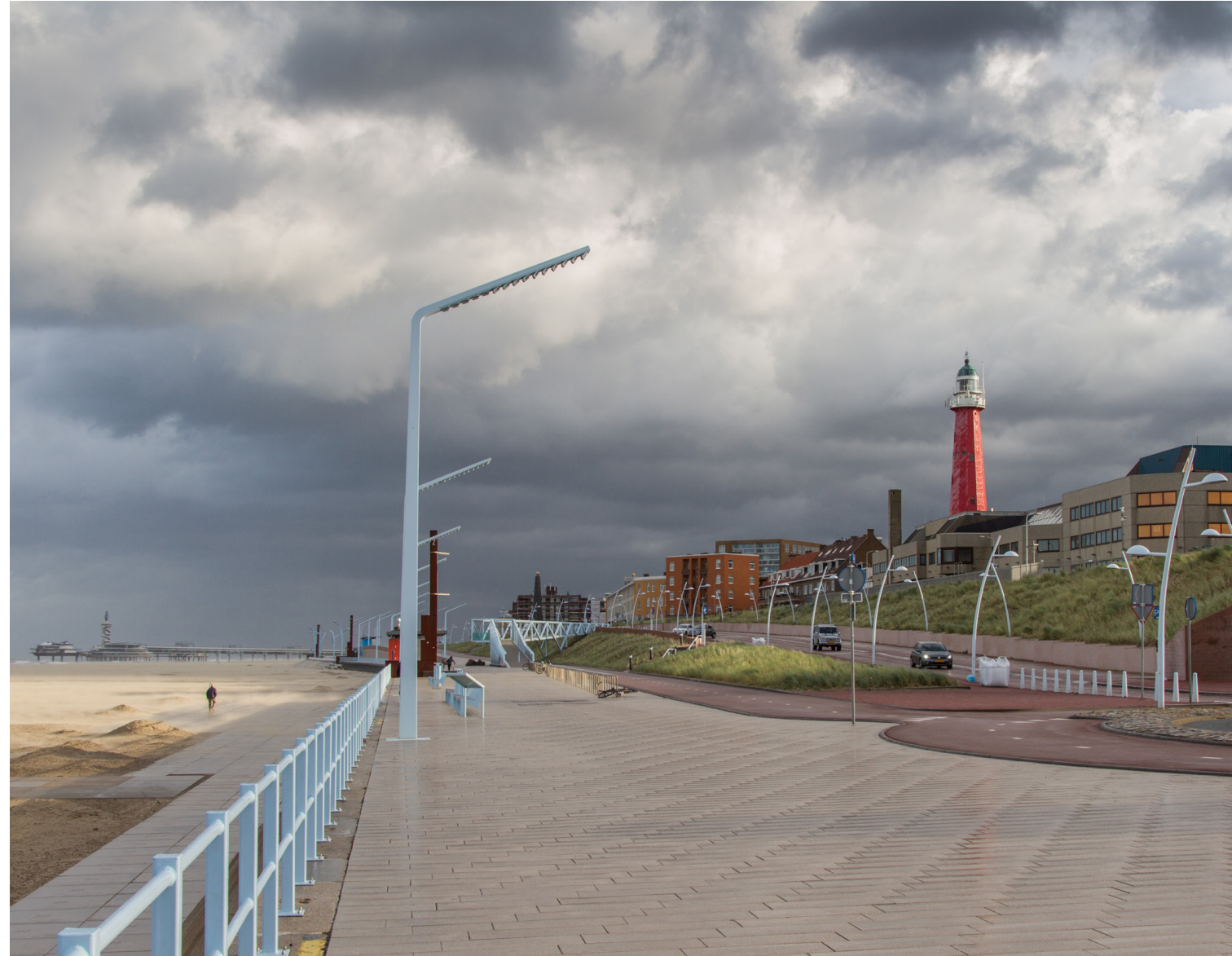
Figure 102. Multifunctional flood defense The Hague- Scheveningen Boule- vard: a dike protected by a widened beach and concealed beneath an undulating pedes-
