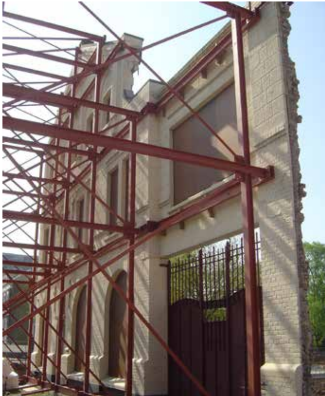
FIG. 3.8 Nieuwe Haven, Schiedam: the facade of a former genever distillery breaks down the volume of a new residential complex. De Roon Architecten, 2007. [FIG. 3.8–3.9]
