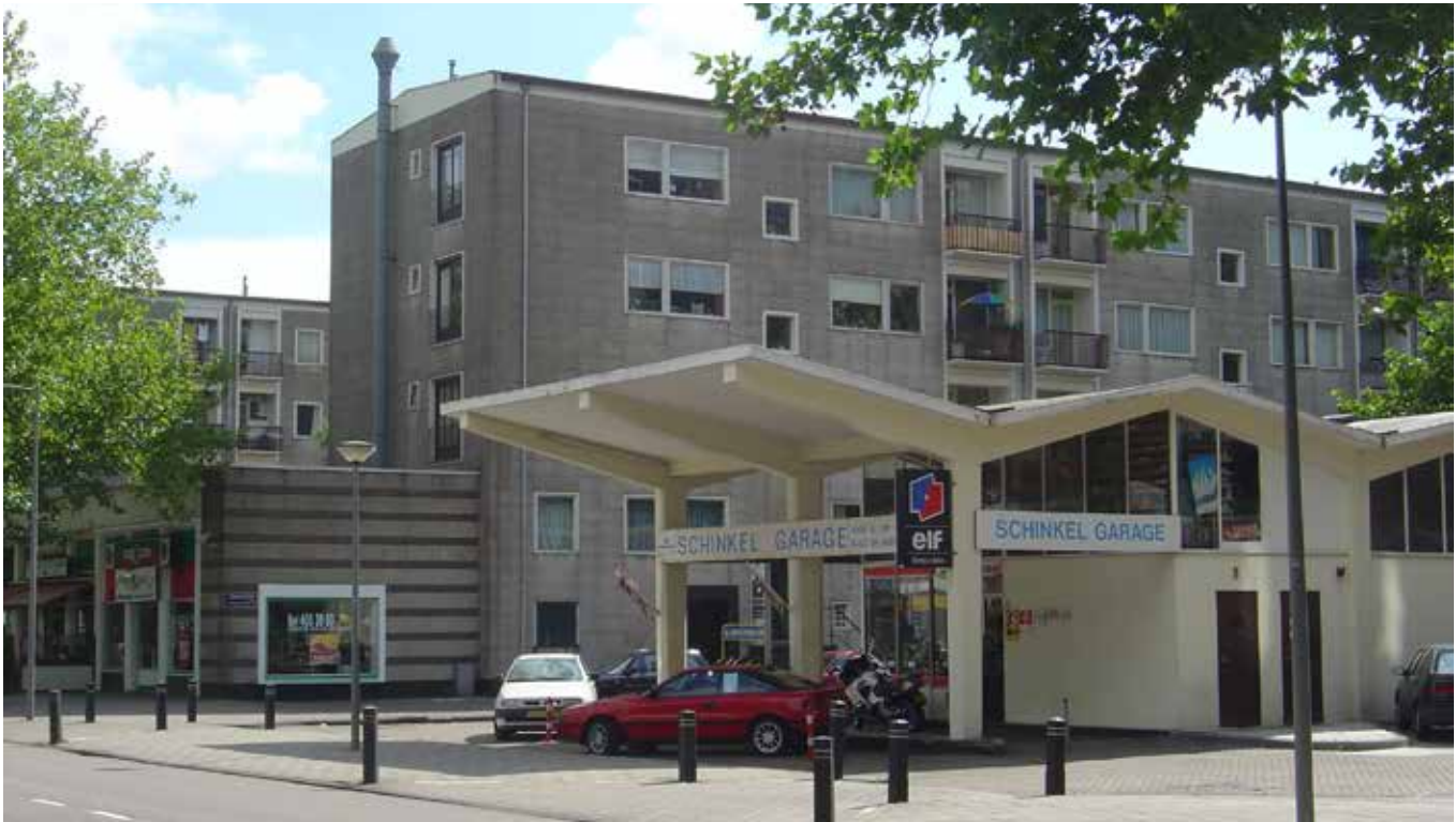
FIG. 1.9 Sloterhof, Amsterdam, J.F. Berghoef (1959). The Nemavo-Airey building system was used to create an ensemble of 14 apartment buildings and 4 towers, with shops, garages and other facilities.
