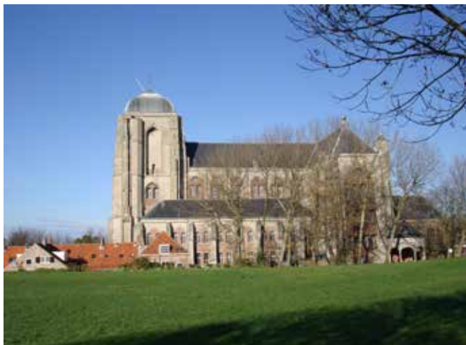
FIG. 1.6 The monument as exceptional building: O.L. Vrouwekerk, Veere.
