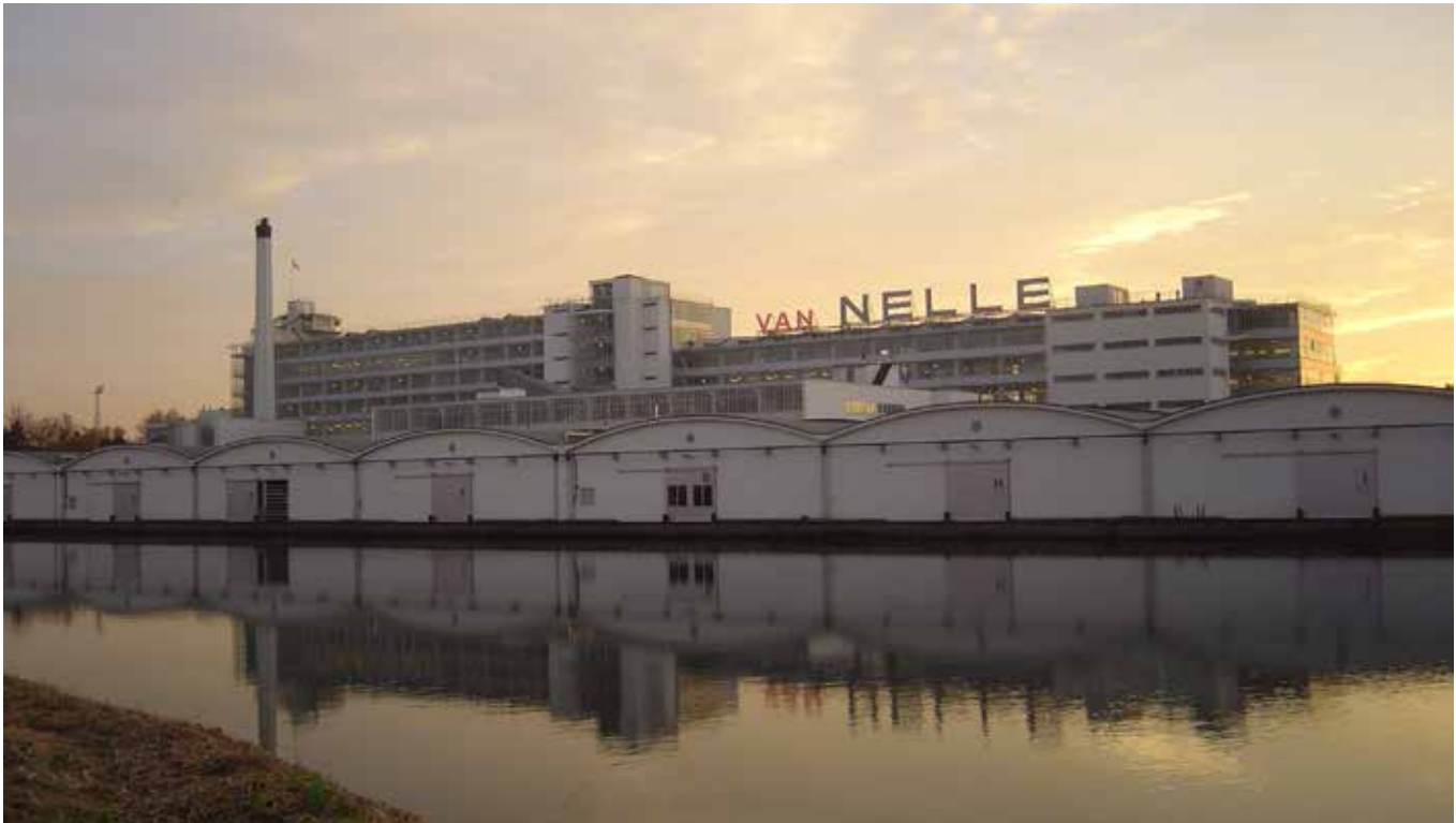
FIG. 3.10 Van Nelle, Rotterdam: the construction of a second façade behind the original façade enabled the strict conservation of the exterior. Wessel de Jonge Architecten, 2004.
