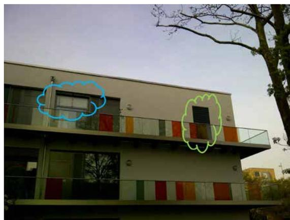
► **Fig. 3:** Building-integrated demonstrators in the façade of BASF's LUMit building: translucent closed element (blue cloud, left) and opaque open element (green cloud, right)
