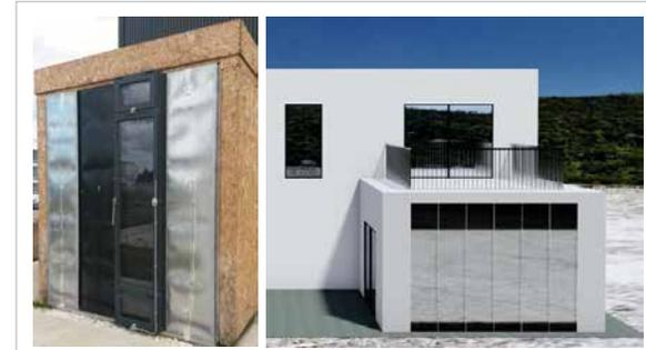
► Fig. 2: EcoSteel panel experimental prototype and virtual prototype integrated in a LSF house.
