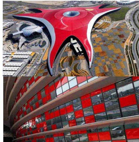
► Fig. 1: Ferrari World Abu Dhabi building is aligned on the north-south axis to maximize shading from the tri-form arms on the primary façade. This has the advantage of reducing solar gain and heat loads within the building itself ([www.e-architect.co.uk](http://www.e-architect.co.uk)). The façade is furnished with solar control glass and individual screen printing. ([interpane.com](http://interpane.com)). (Photo top: Wikipedia.com, bottom: Interpane.com)
