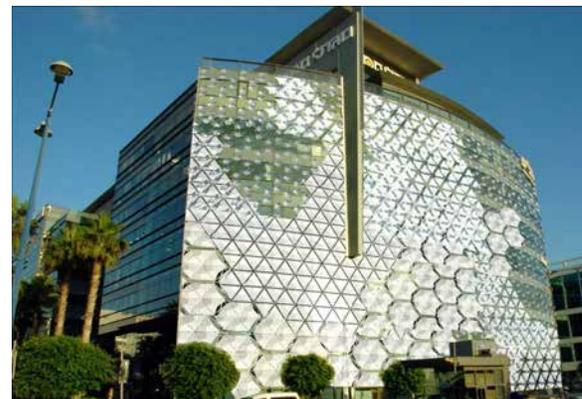
► Fig. 3: The western façade of Migdalei Tamam with the proposed shading solution, using smart materials for the actuating function, according to climatic and functional requirements.
