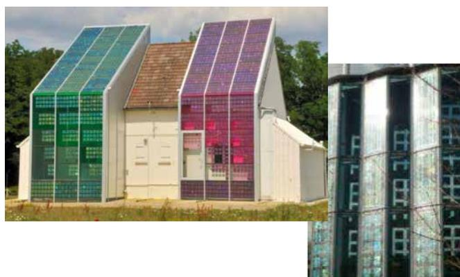
► **Fig. 2:** Double-skin prototype for detached houses (ETNA Test house – EDF R&D) - Pleated façade prototype for office buildings (HBS-Technal)
