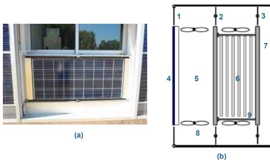
Fig. 1: (a) BIPV/T-PCM system in a south façade of an office in Solar XXI; (b) Scheme of the BIPV/T-PCM system.
