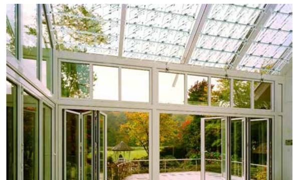
▶ Fig. 3: SolarSwing Energy® in the roof of a glazed sunspace
