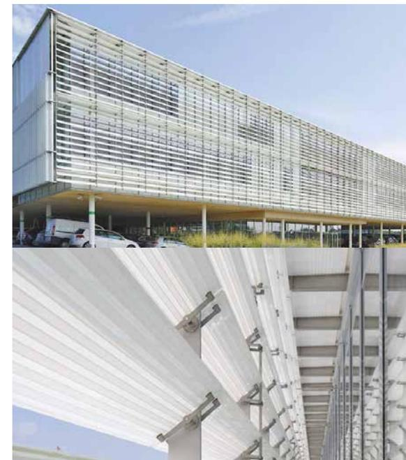
► Fig. 2: Head office of AGC - Glass Europe. The sunshades of this building adapt automatically to the sun angle. Diffused natural light can still enter the building, because the sunshades are treated and printed with alternative bands of white. (<http://www.domusweb.it>)
