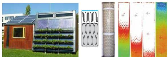
► Fig. 5: Self sufficient building (left) with integrated decentralized ventilation unit (centre) and active natural heating system with air vacuum tube SC and PCM storage (right).
