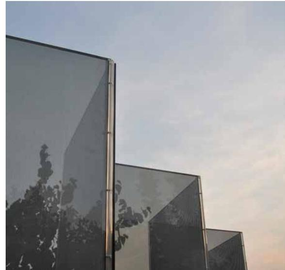
► **Fig. 1:** Final full-scale prototype of the folded reinforced glass facade panel system.
