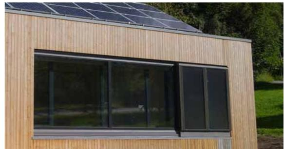
▶ **Fig. 2:** Double skin windows with ventilation features, façade integrated solar thermal collectors and roof integrated PV panel installed on the ZEB Living Laboratory
