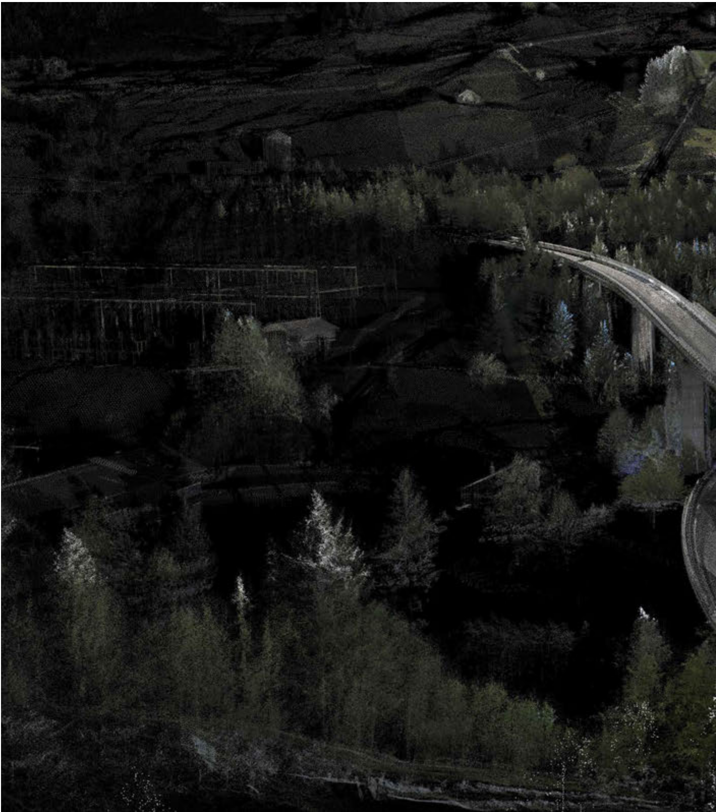
FIGURE 5.14 True-colour 3D laser scan of a landscape section through infrastructures near Airolo (Switzerland) combining terrestrial laser scanning and point cloud technology (image courtesy of Pascal Werner, Chair of Professor Girot, ETH Zurich, 2015)
