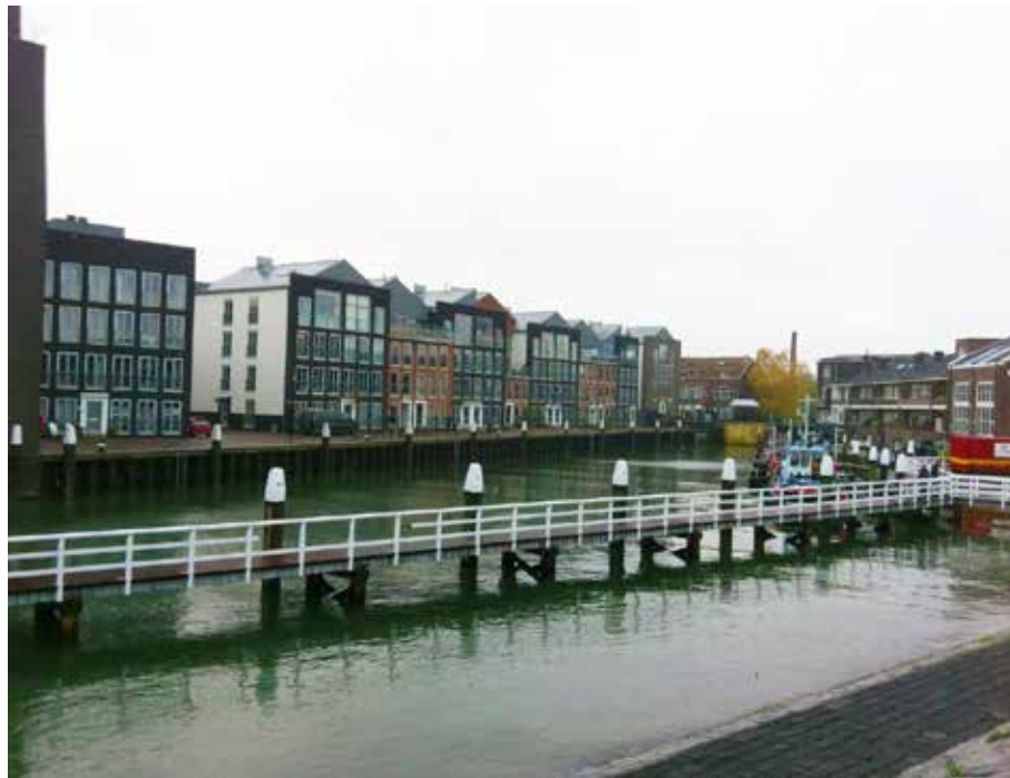
FIGURE 8.5 New housing project in Dordrecht
