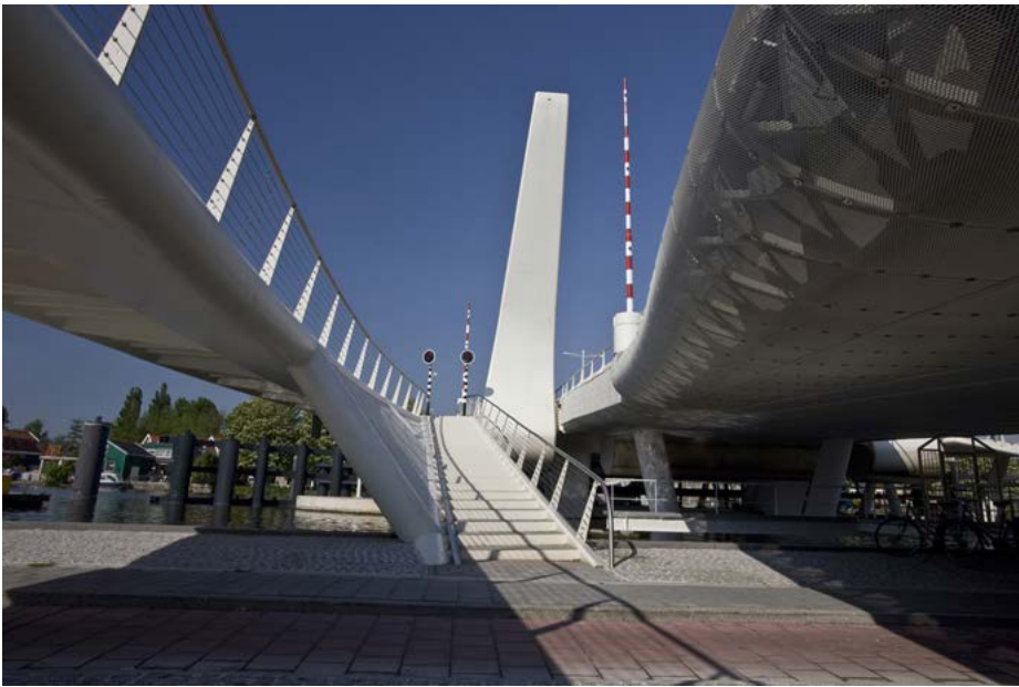
Figure 6 The Prins Bernhard Bridge a multi-layered bridge with access to the river quays, 2007 (source: Joris Smits)
