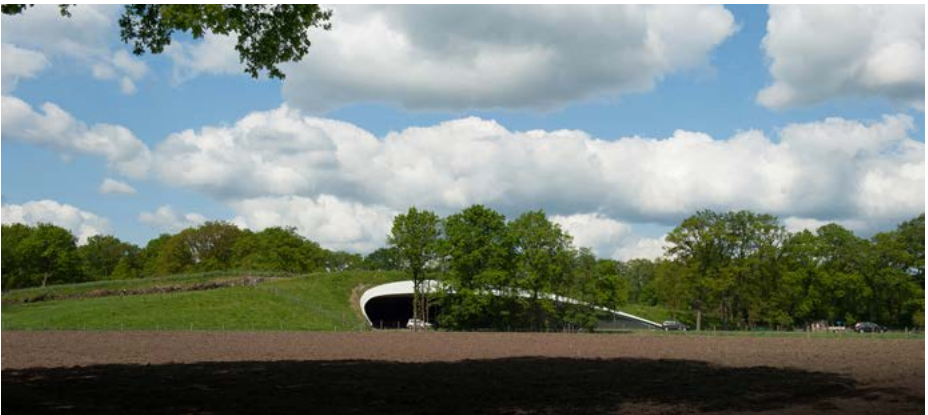
Figure 16 The wildlife crossing at Rijssen. Nature has the supremacy, in the form of soil and vegetation; the road is just a perforation of the earth, a guest that is temporally tolerated underneath it (source: Joris Smits)
