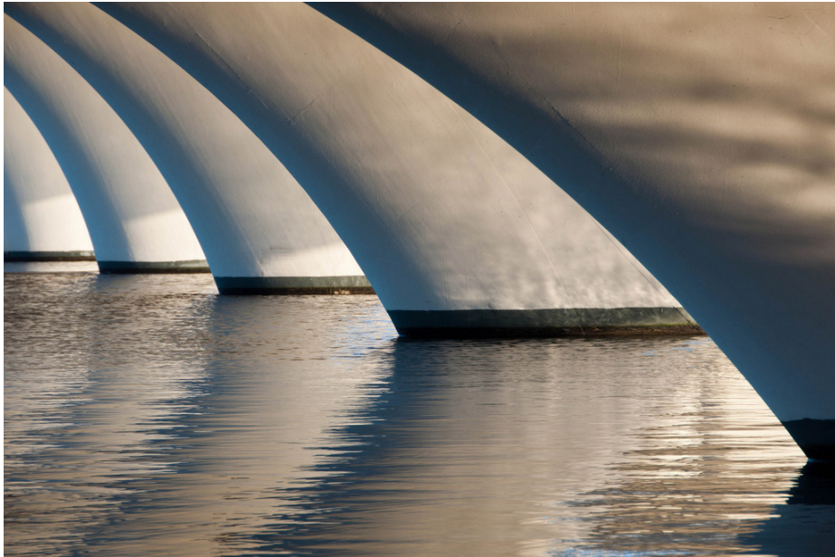
Figure 10 Ambient light underneath the bridge increases by the use of a void between the decks (source: Joris Smits)
