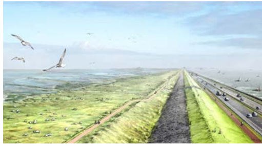
Figure 16 Redesign of the Dutch Closure Dam by landscape architect Hosper (Lammers, 2009). The green land to the left is currently not there; vegetation is to grow over artificial sand nourishments of several metres high. The concept is promoted by the NGO Natural Climate Buffers , in which the major Dutch nature conservation organisations collaborate. The NGO frequently uses the terms natural safety and natural flood defences in their communication, for example towards the Delta Program (SNK, 2014). Also see figure 19
