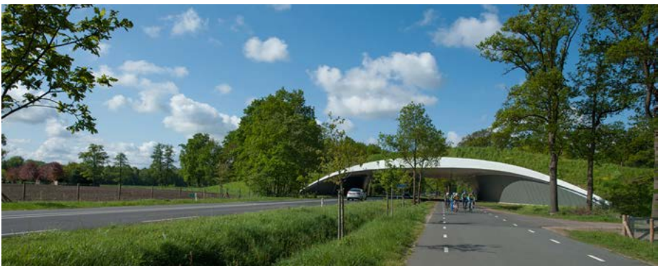
Figure 18 'Lifting the carpet' leaves a slit-like opening underneath the green structure. The low parts of the slit are filled with solid abutments with a set back from the edge. They are materialised in a dark grey colour in order to blend with the ground rather than with the crescent edge. This results in the impression of one long continuous edge (source: Joris Smits)
