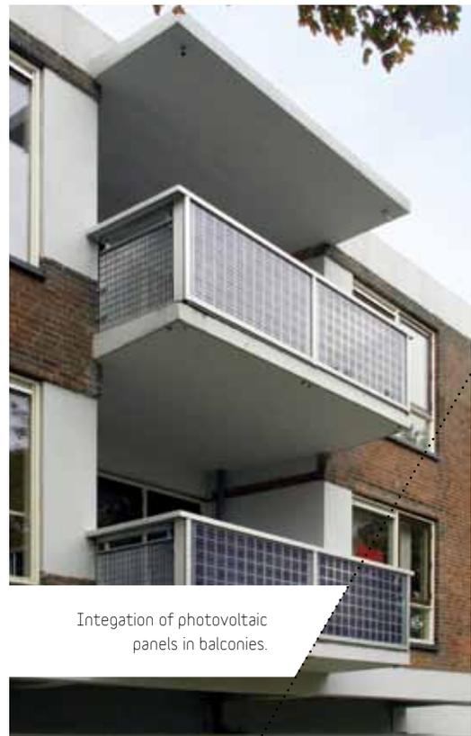
Integration of photovoltaic panels in balconies.
