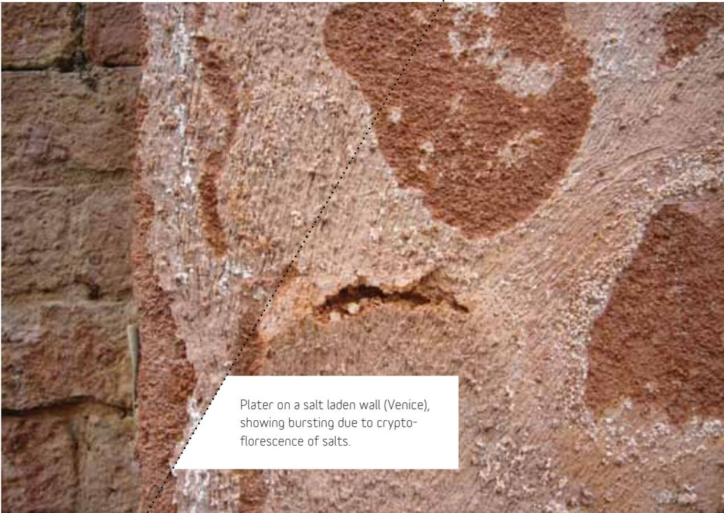
Plater on a salt laden wall (Venice), showing bursting due to crypto-florescence of salts.
