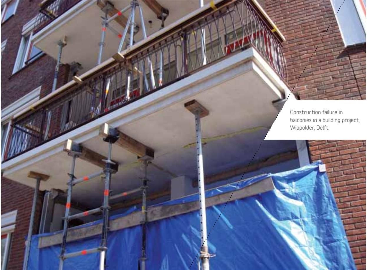
Construction failure in balconies in a building project, Wippolder, Delft.
