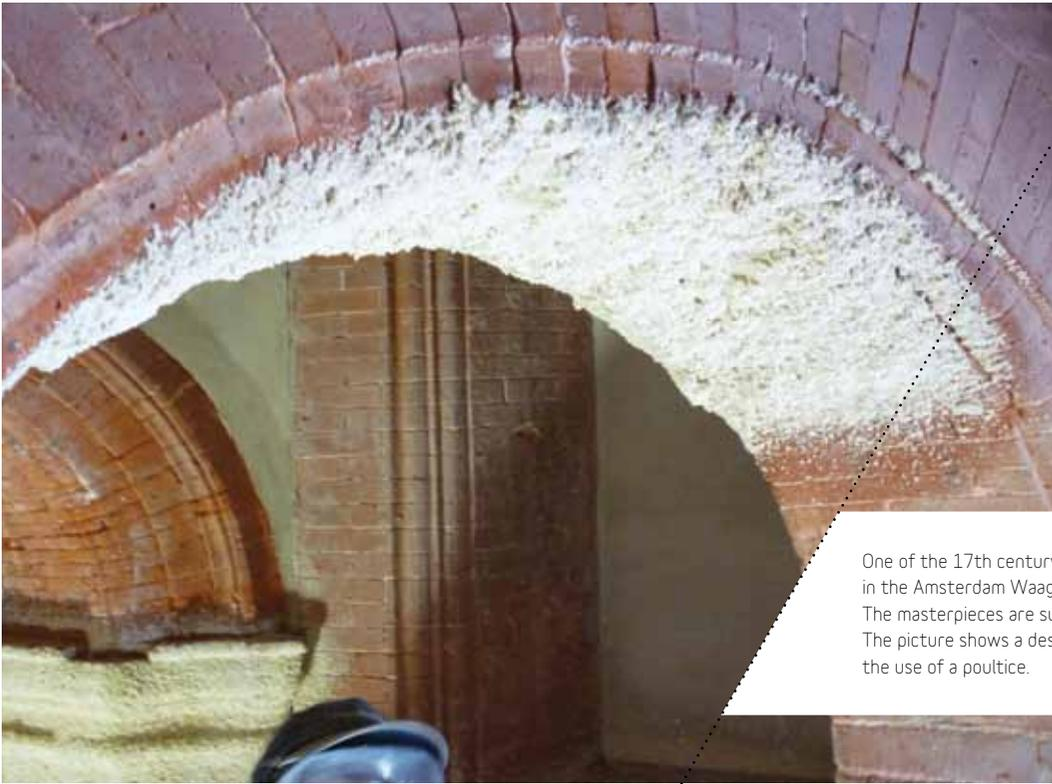
One of the 17th century masonry masterpieces in the Amsterdam Waag building. The masterpieces are suffering severe salt decay. The picture shows a desalination operation with the use of a poultice.
