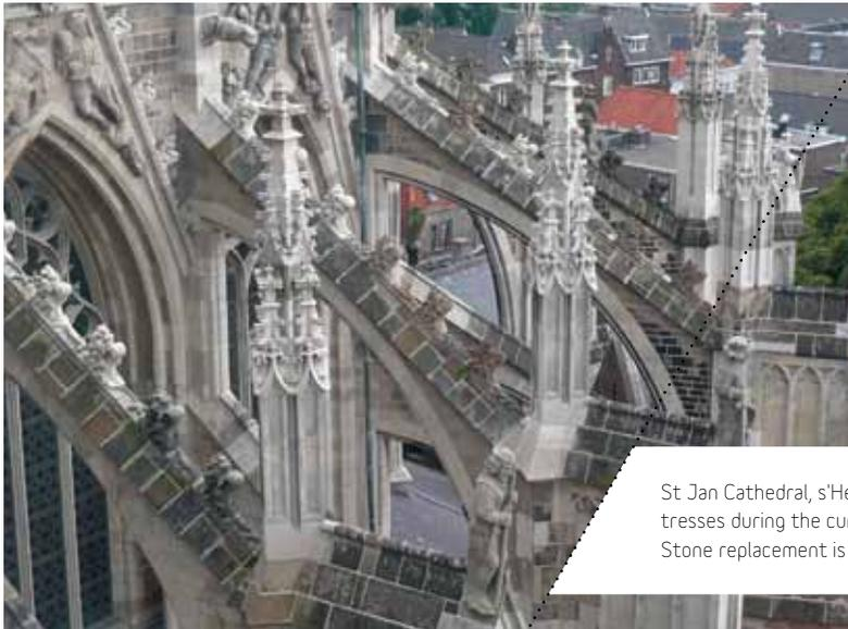
St Jan Cathedral, s'Hertogenbosch. View of flying buttresses during the current restoration campaign (2009). Stone replacement is visible in the light coloured elements.
