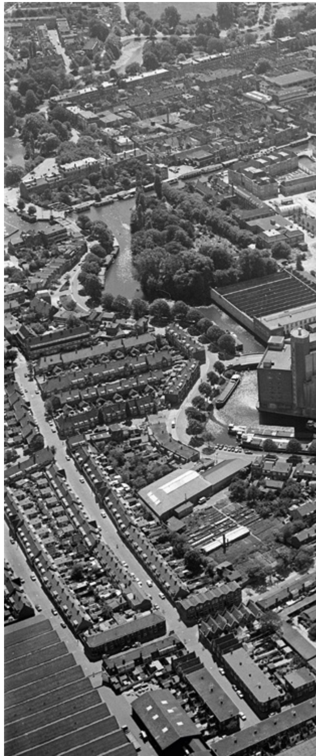
1976 Aerial photograph of south Havenwijk after demolition
