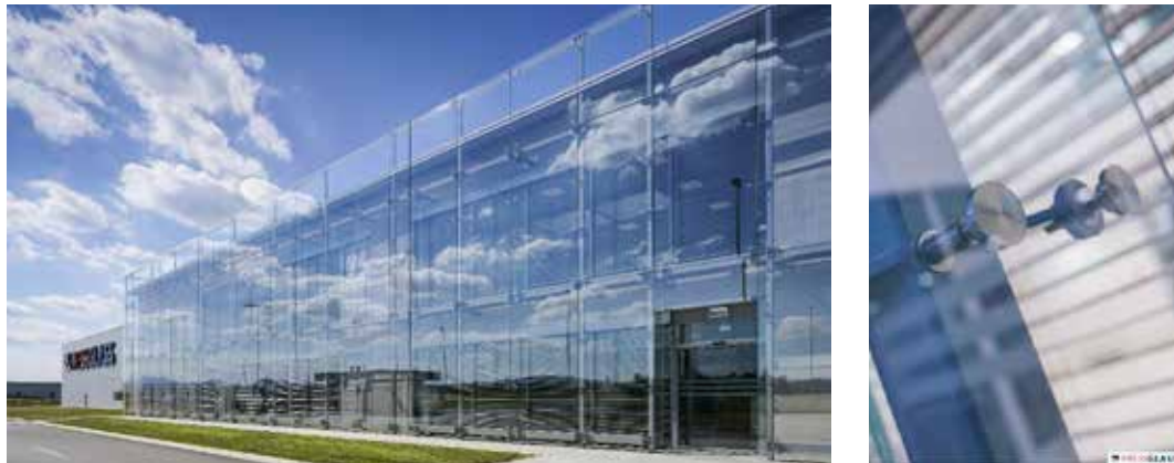
FIG. 1 Left: Example of TSSA application (PressGlass office, Croatia). Right: detail showing the optical clarity of the silicone film
